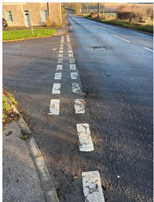
16 – White lining has deterioration, to receive heavy traffic.
