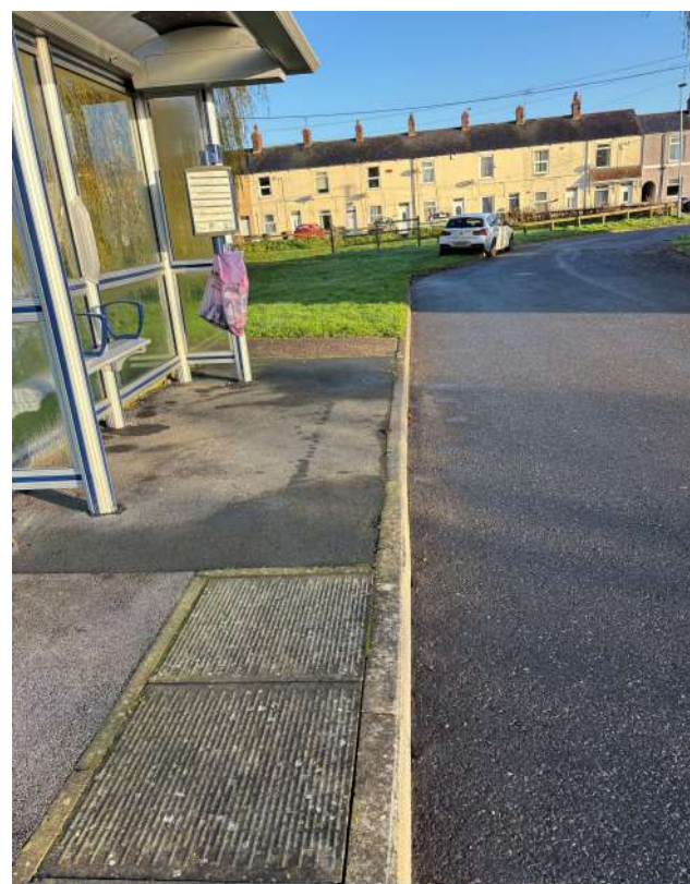
12 – Kerb line at bus stop in good condition, minor chipping.
