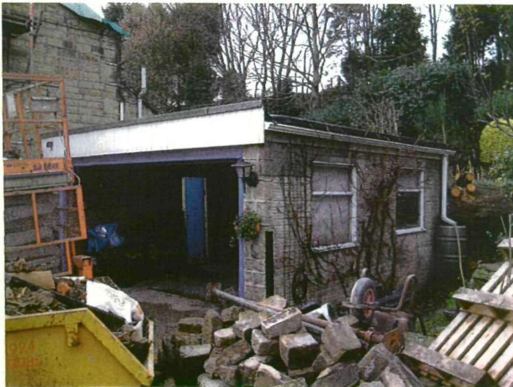
6. Existing single storey flat roofed double garage to be demolished
