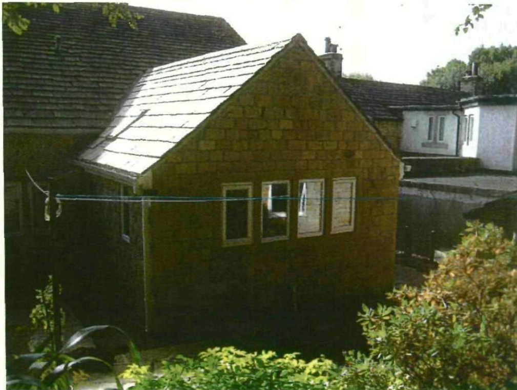
4. Existing single storey extension to the rear
