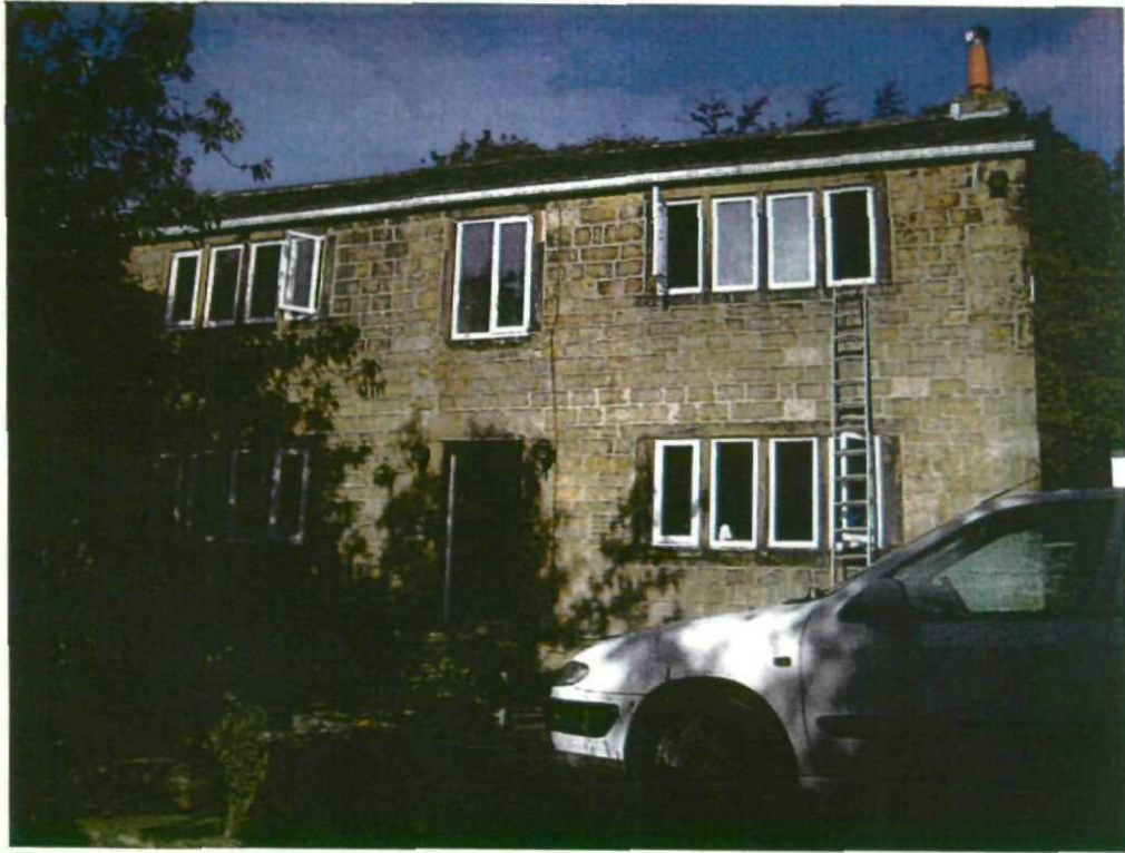
1. Front (south) elevation to the existing house
