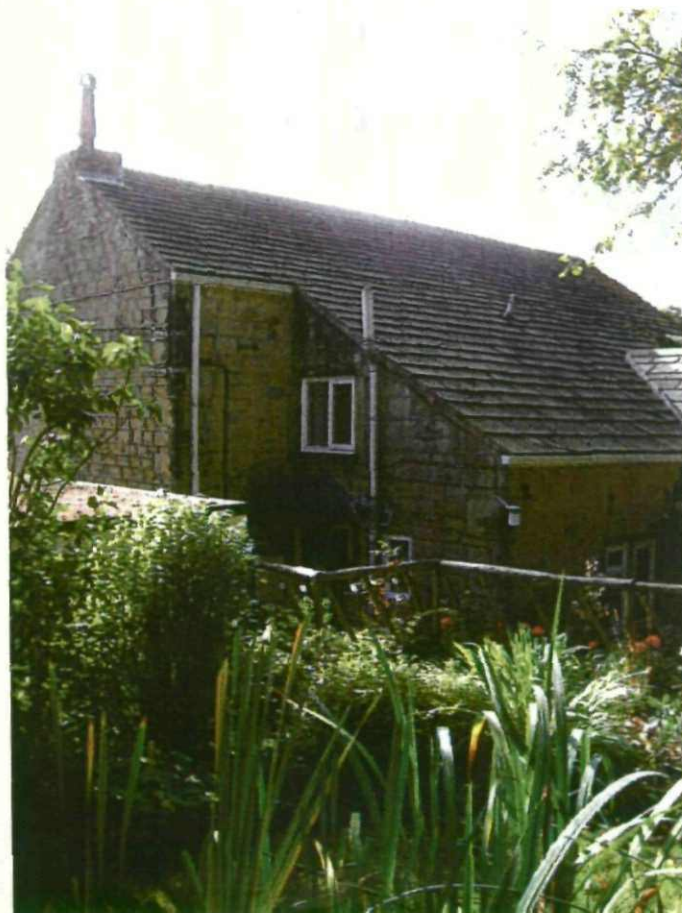
2. Rear elevation (north) of the existing house
