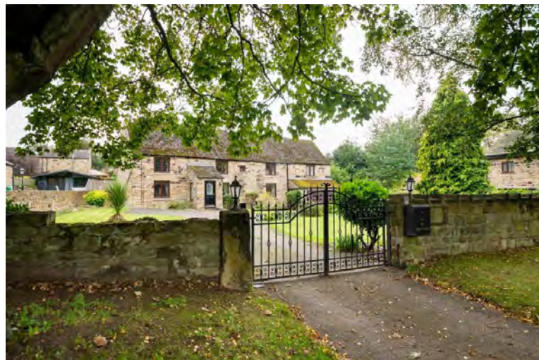
View Of Hirst Cottage From Chapel Lane
