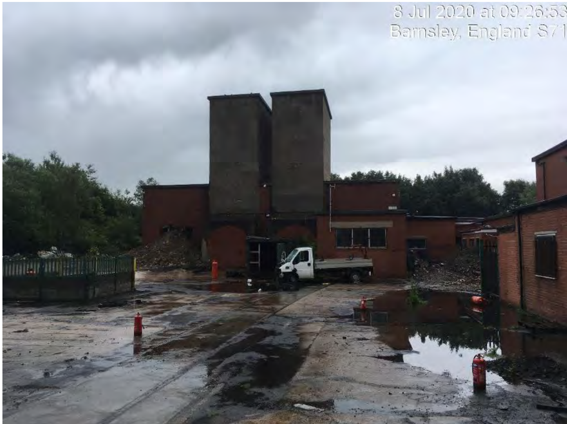
Photo 13: Engineering Yard east of the Coal Stockyard
