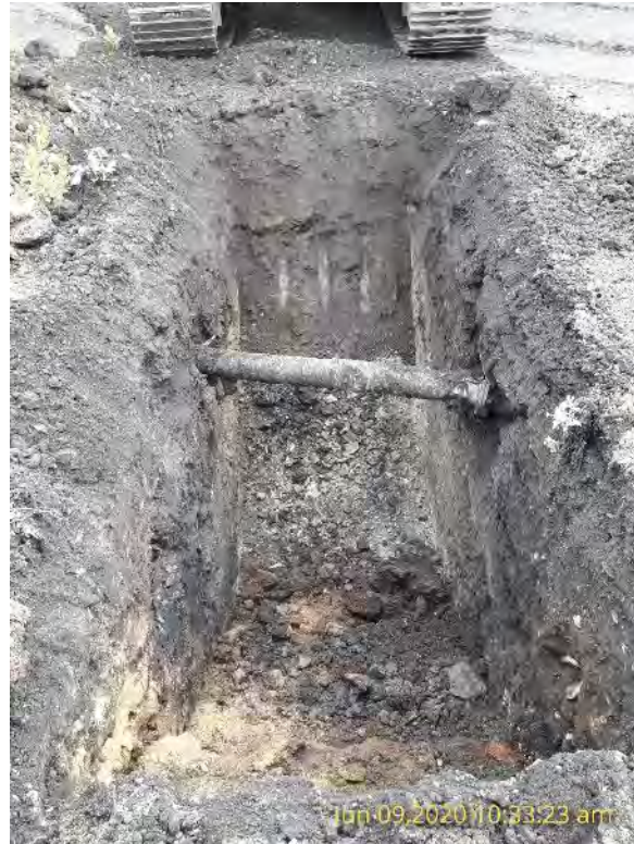
Photo 33: TP61 Showing underground infrastructure in Coal Stockyard
