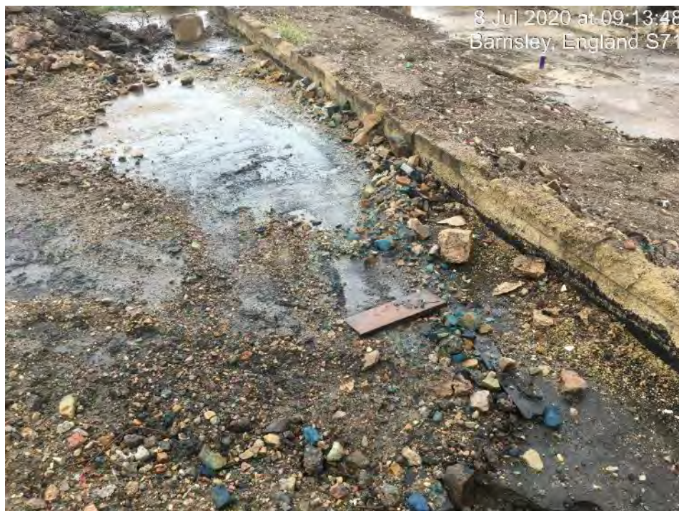
Photo 6: Blue staining likely to be associated with cyanide impact.
