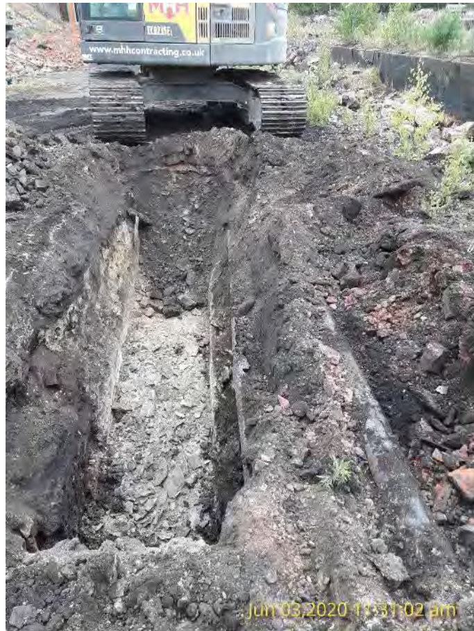
Photo 29: TP28 in Production Area showing underground infrastructure
