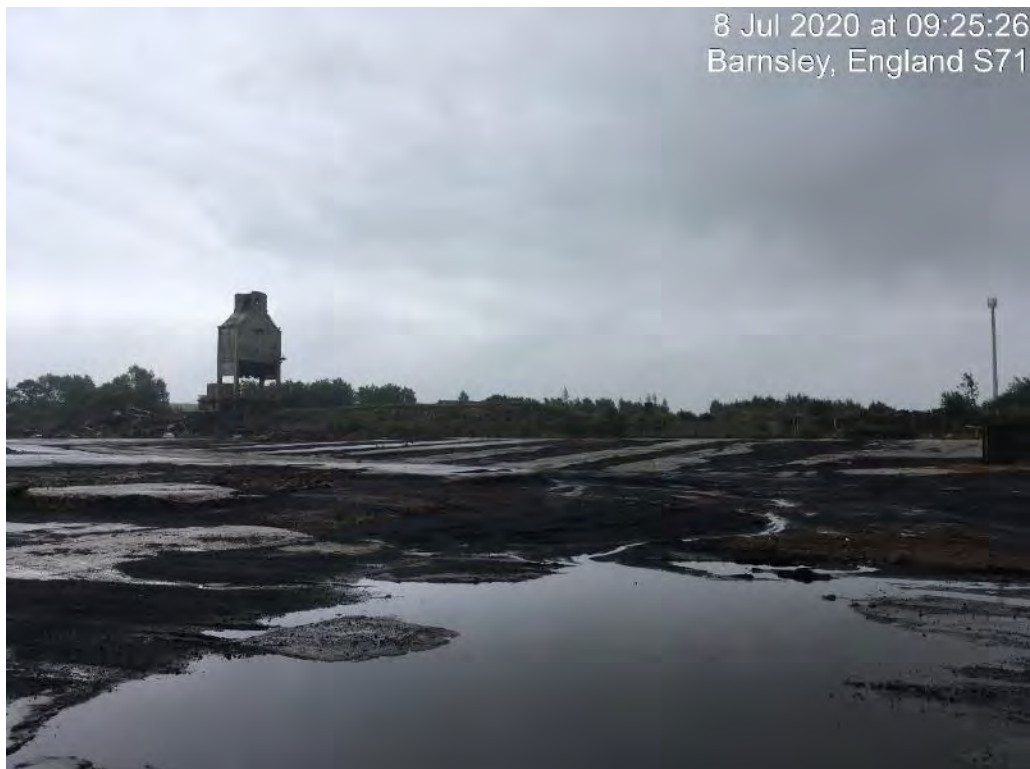
Photo 10: Coal Stockyard looking North towards Production Area
