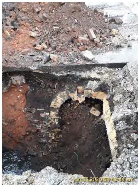
Photo 18: TP24 showing identified tunnels
