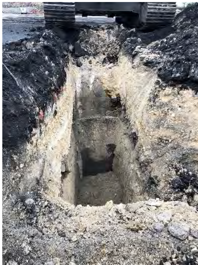
Photo 24: TP70 showing concrete wall
