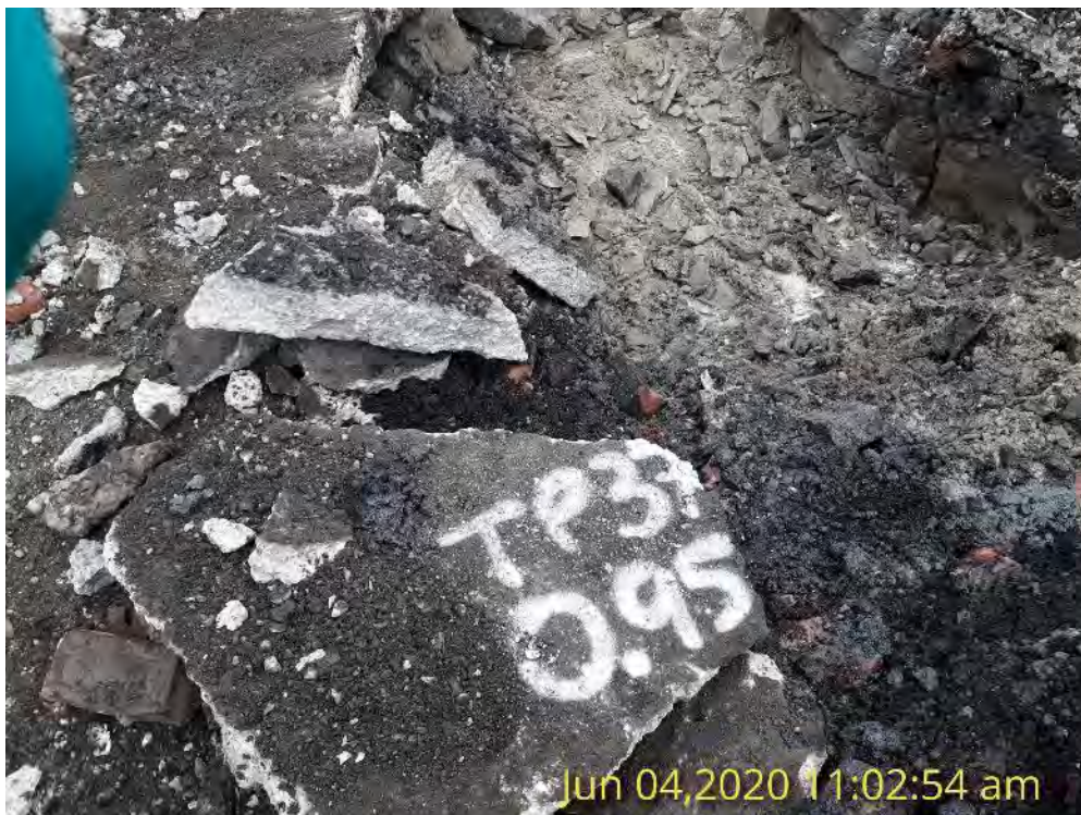
Photo 30: TP37 in Production Area showing coal tar impacted soils above grey sandstone bedrock
