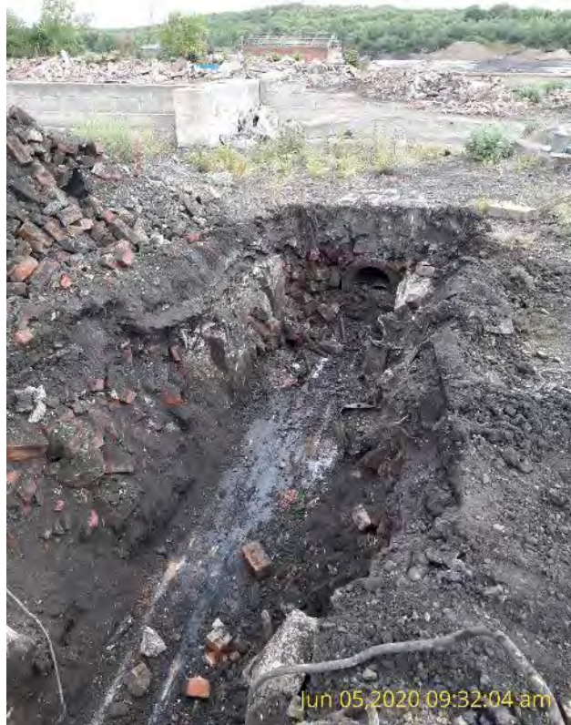
Photo 21: TP49 showing concrete base and side with large diameter pipe
