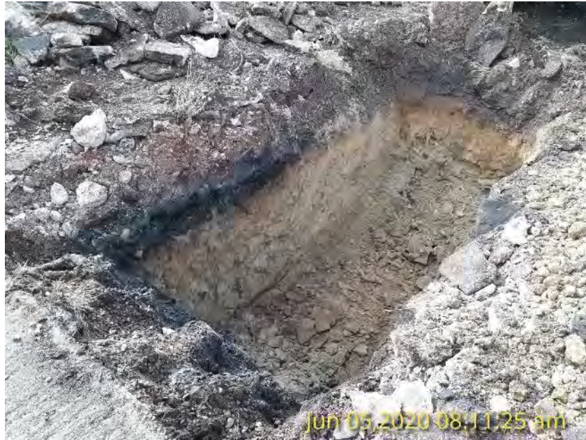
Photo 31: TP44 in Production Area showing shallow tar impact above bedrock.
