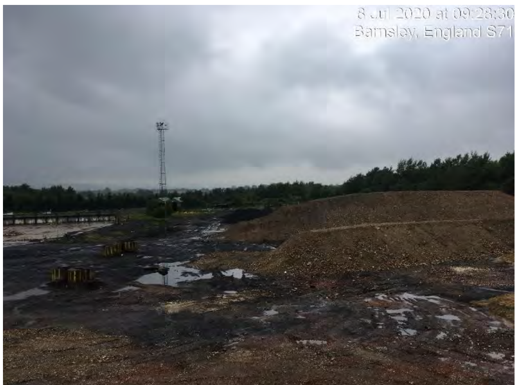
Photo 12: Northern area of the Coal Stockyard with stockpiled material. Concrete rings are location of manholes for a sewer.
