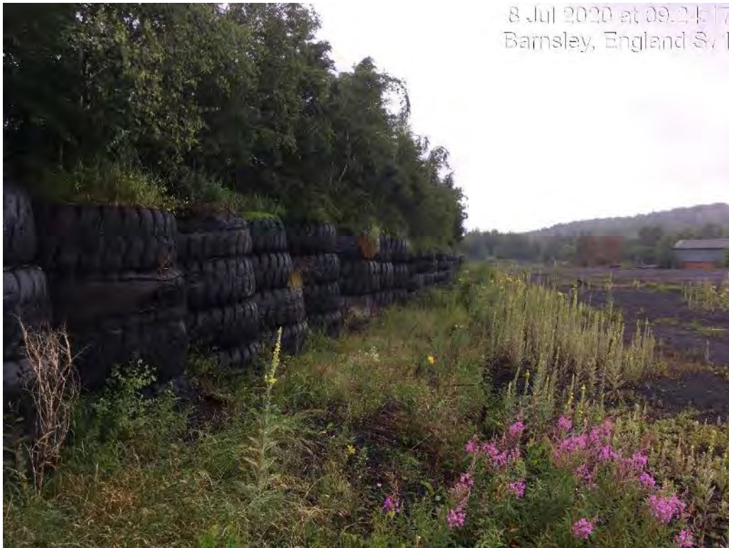
Photo 11: Looking north in Coal Stockyard along the western boundary denoted by a tyre wall.
