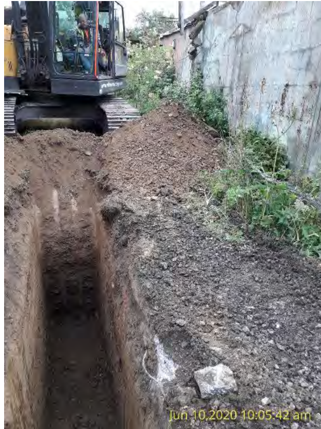
Photo 35: TP72 in the Southern Area in mudstone
