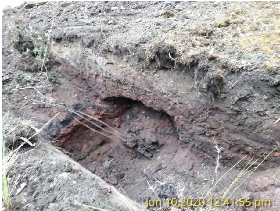
Photo 23: TP77 potential railway tunnel.
