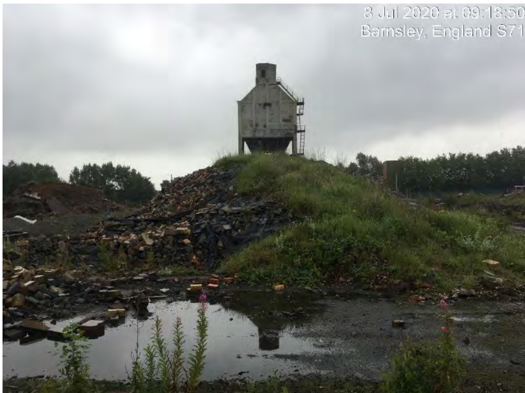
Photo 8: Mound of Silica brick deposited west of the remaining tower.
