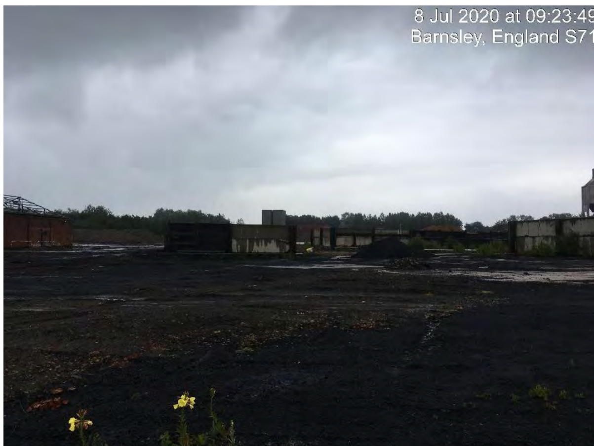
Photo 15: Coal Stockyard looking west from the east with thin coal breeze surfacing.
