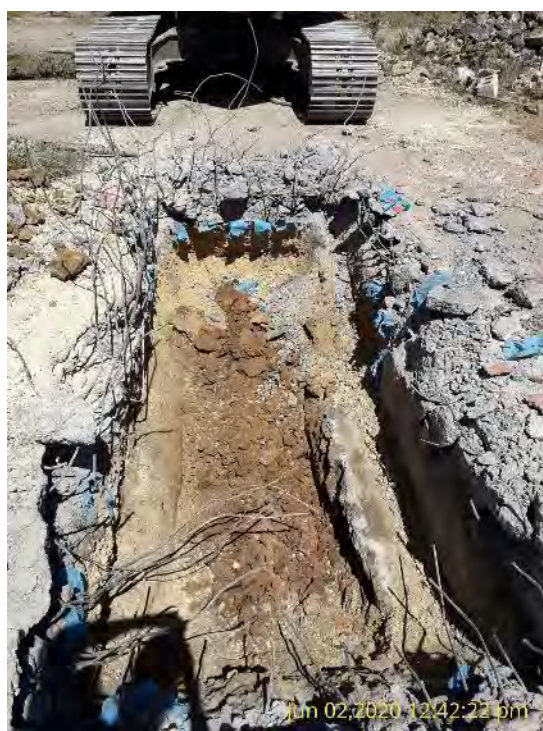
Photo 16: TP18 in CHP area showing reinforced concrete
