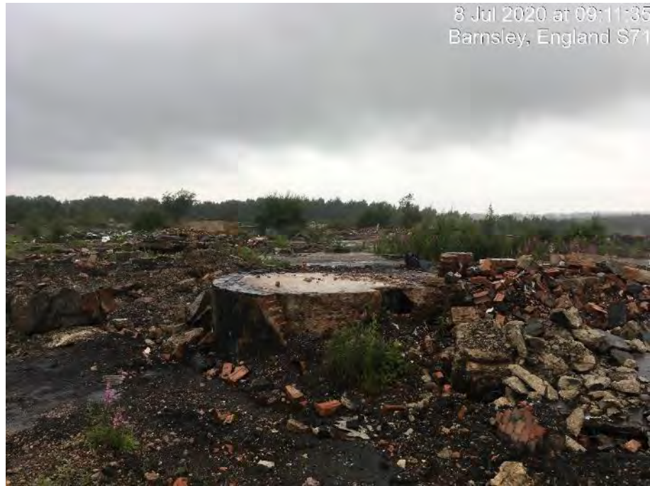
Photo 5: Looking west over the former production area. Concrete structures still present with coal tar staining.
