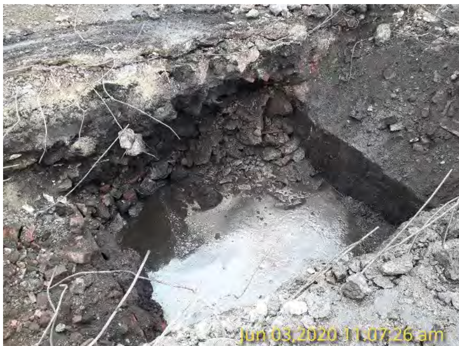
Photo 28: Tar impacted water in the Production Area
