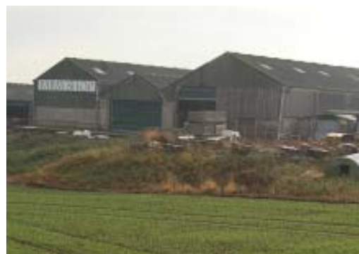
Existing Farm Sheds
