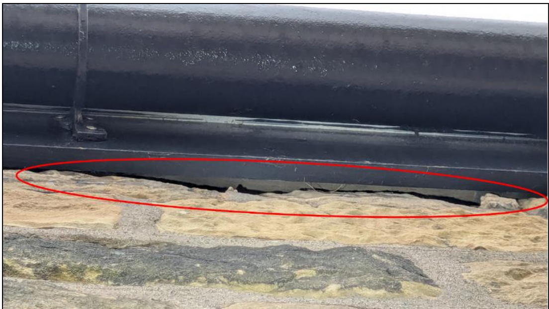
Plate 9. Gap behind fascia board on northeast elevation of Daisy Cottage
