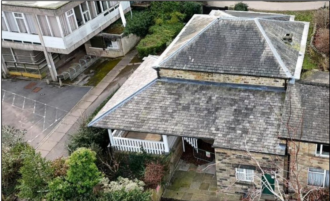
Plate 6. Gun Room, viewed from northeast
