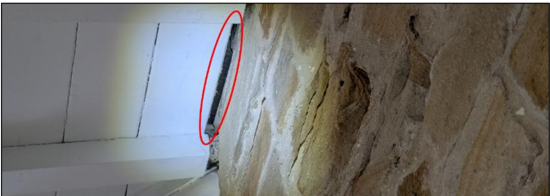
Plate 12. Gap at top of sarking on underside of veranda roof, potentially allowing bats access to crevice space behind flashing.
