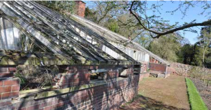
Existing North Range Glass House
