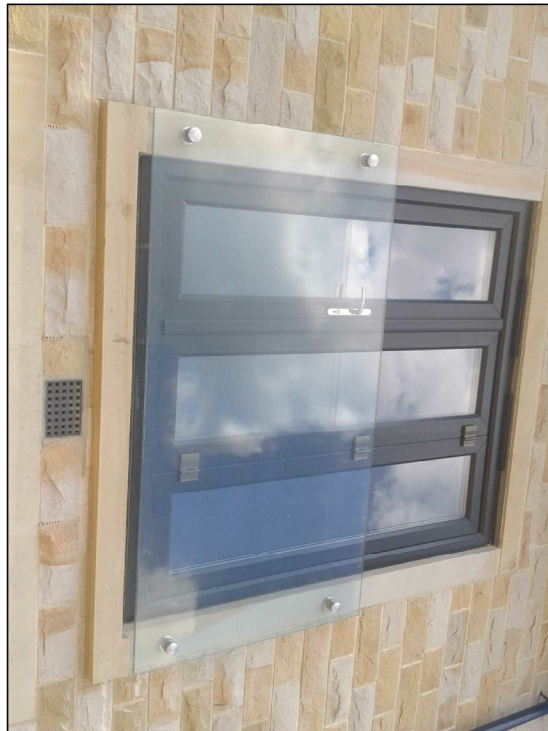
FRAMELESS GLAZED GUARDING TO FIRST FLOOR DOORS
