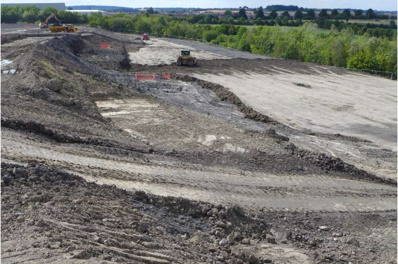
Photograph No 6: taken on 01 September 2022 – Continued work on increasing the levels in the External Yard Area, with monitoring rod in the centre of the rolled area.
