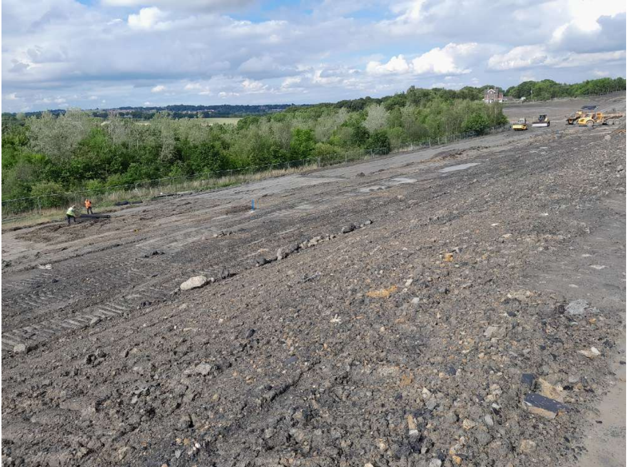
Photograph No 2: Taken on 23 August 2022 – Monitoring rod (blue tubing) locations in background on proposed External Yard Area.
