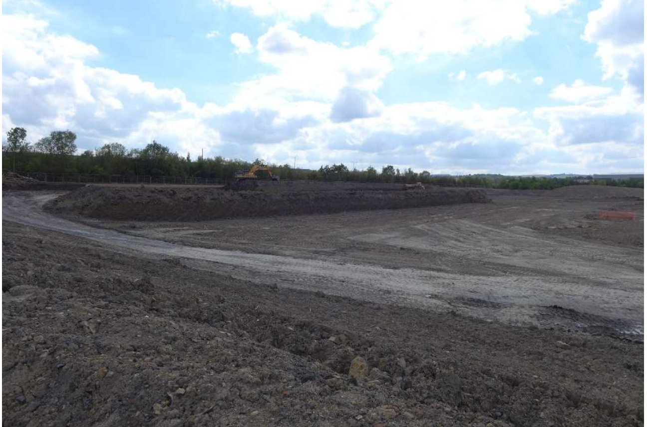
Photograph No 7: taken on 05 September 2022 – Removal of surcharge for engineered fill.
