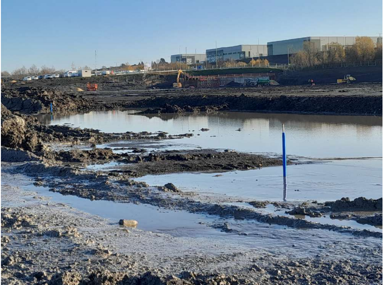
Photograph No 9: taken on 28 November 2022 – Monitoring visit showing monitoring rods in-situ after raising of ground levels.
