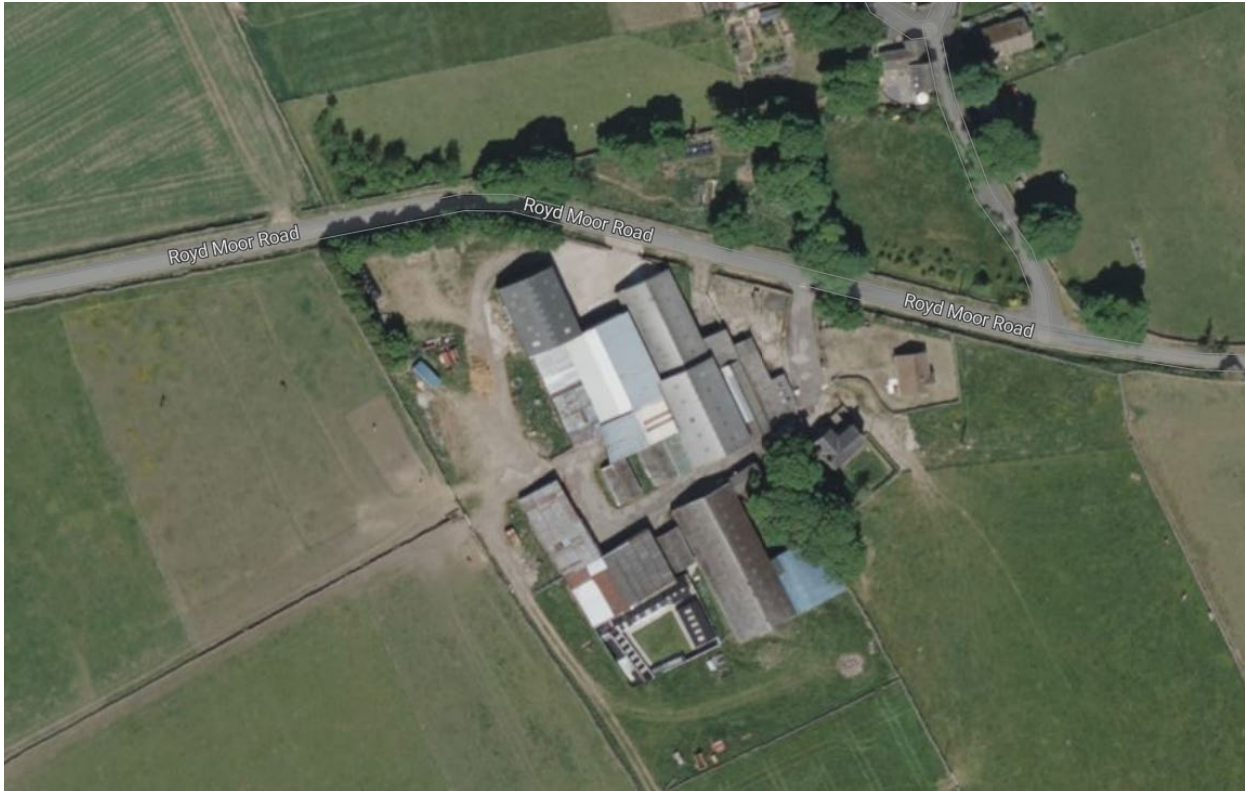
Aerial view of site
