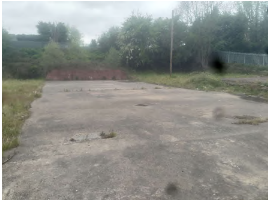
Northern section of site
