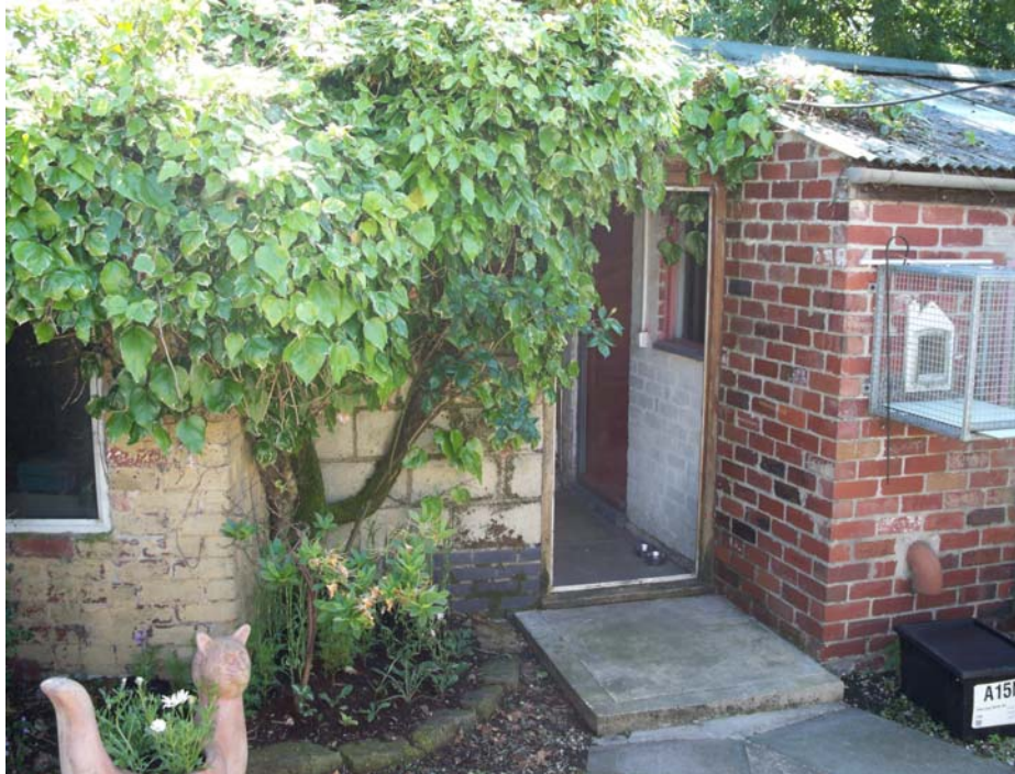
Entrance to Cattery (storage sheds to left)
