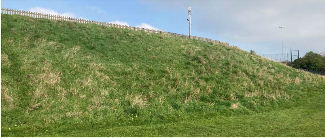
Figure 1-4: From west of site looking west towards the slope and off-site running track
