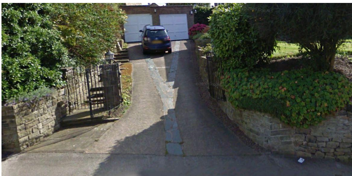
EXISTING SITE ENTRANCE AND DRIVE
