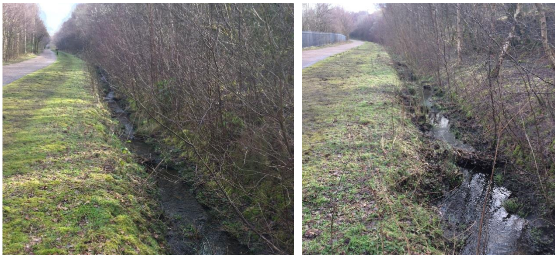
Plates 3 and 4: Existing ditch - typical profile and width (looking eastwards)
