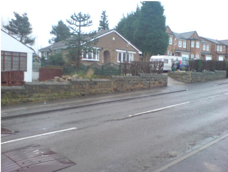
Existing bungalow to the South of the Site
