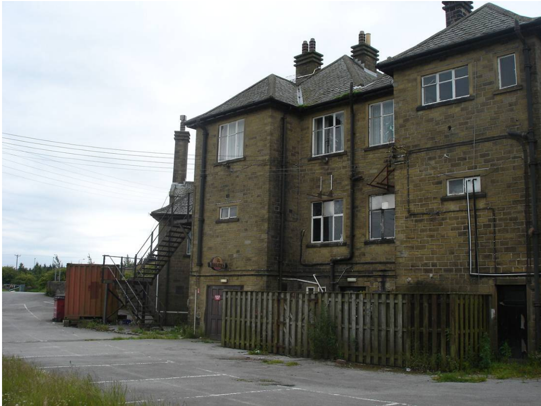
11. Rear elevation - north east, looking south.
