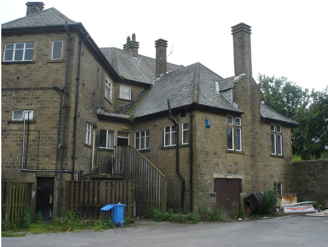
12. Rear elevation – north, looking south west.
