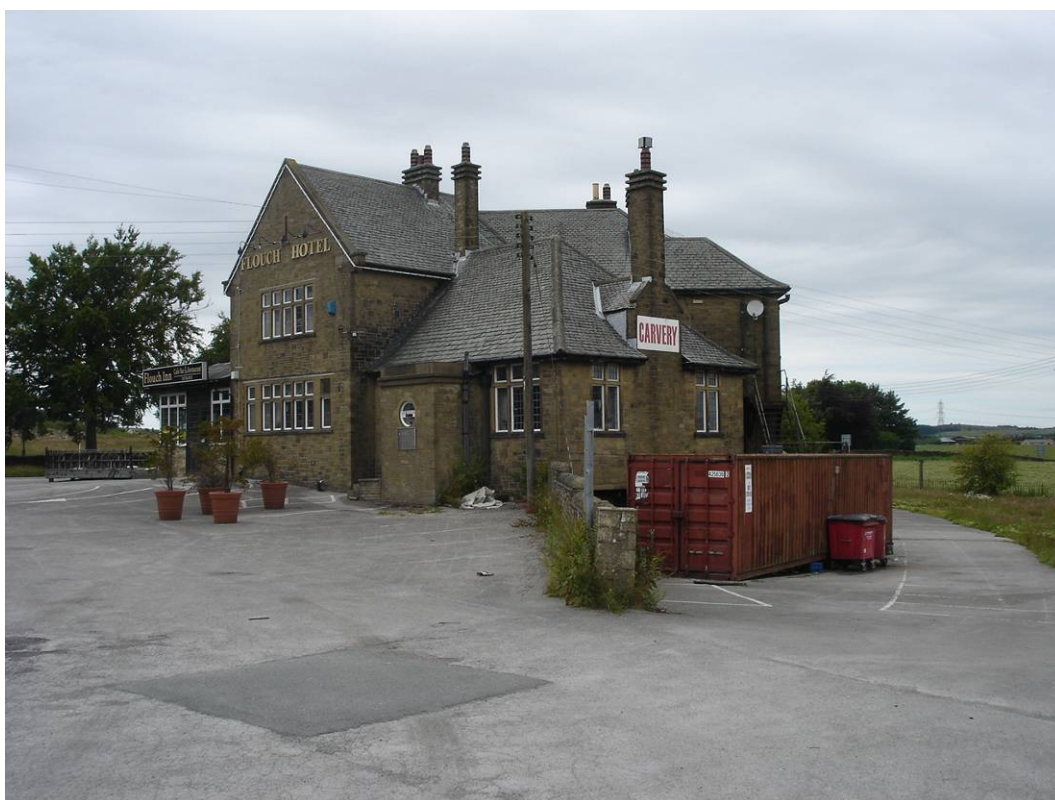
08. Flouch Hotel from south east access.
