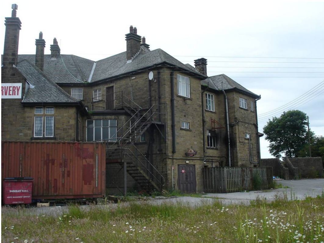
10. Rear elevation - north east, looking north.
