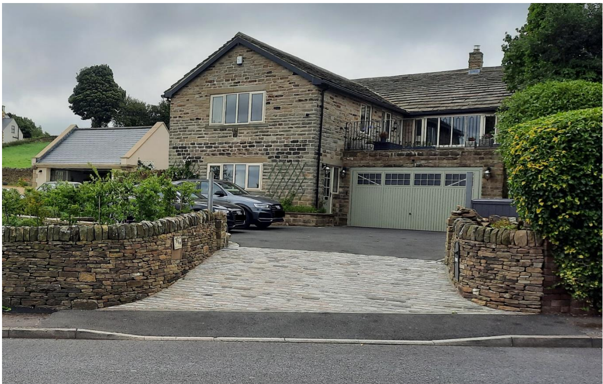
Photograph 6 – No. 268 Barnsley Road
