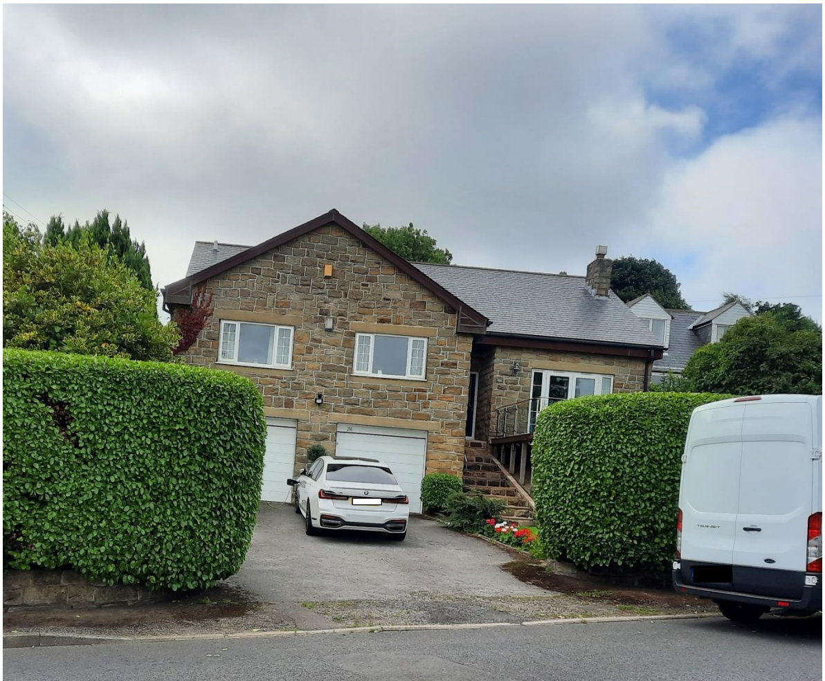
Photograph 5 – No. 266 Barnsley Road
