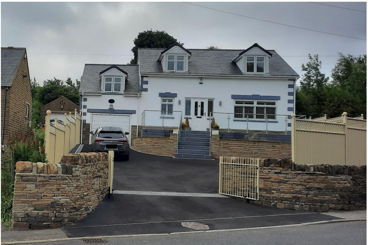
Photograph 4 – No. 262 Barnsley Road
