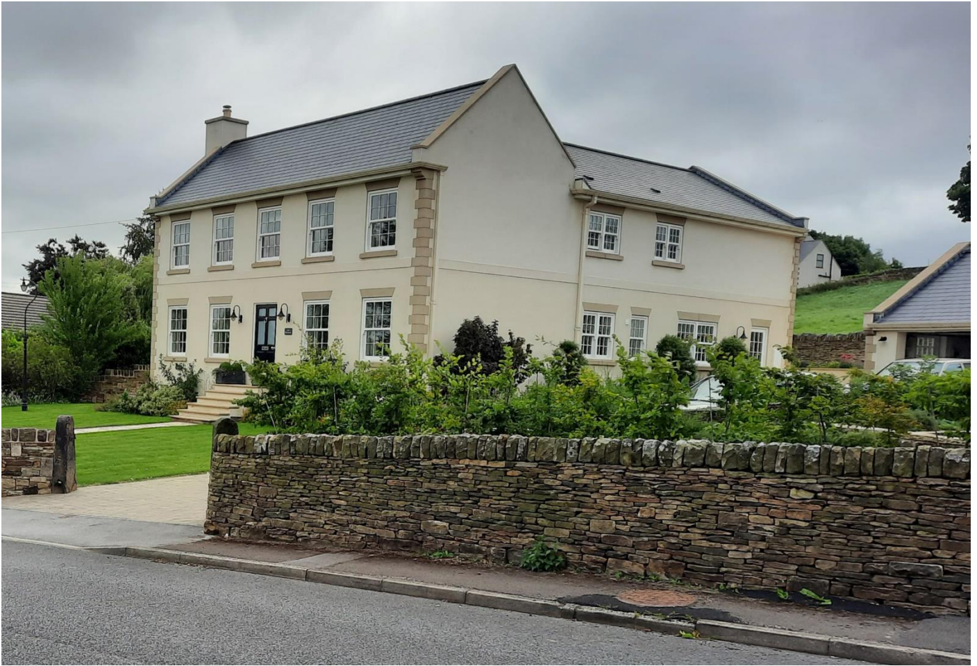
Photograph 7 – No. 270 Barnsley Road
