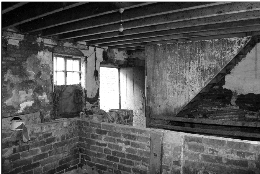
Appendix 2.28: View of the interior of Room G1, Building A , looking south-east
