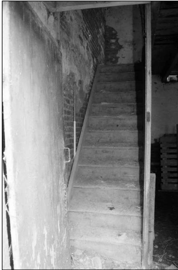
Appendix 2.37: View of the staircase in Room G1, Building A, looking west
