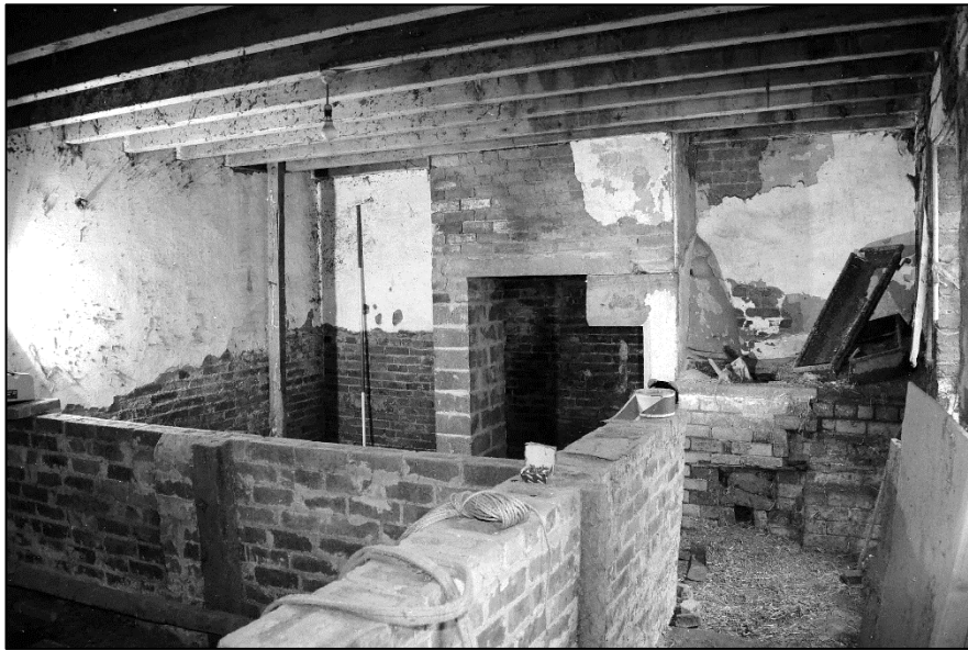
Appendix 2.27: View of the interior of Room G1, Building A , looking north-west
