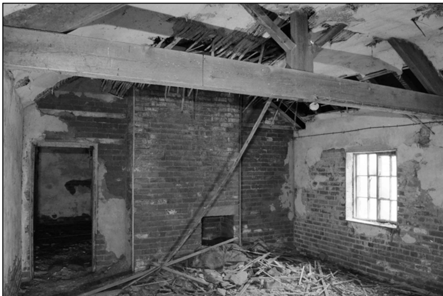
Appendix 2.38: View of the interior of Room F1, Building A, looking north-east
