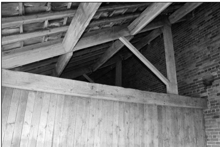
Appendix 2.36: View of the truss above the partition between Rooms G4 & G5, Building A , looking north-east
