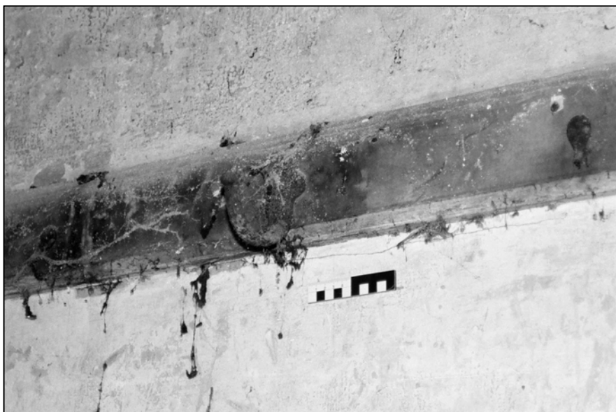
Appendix 2.32: View of tack hooks on the west wall of Room G2, Building A , looking south-west
