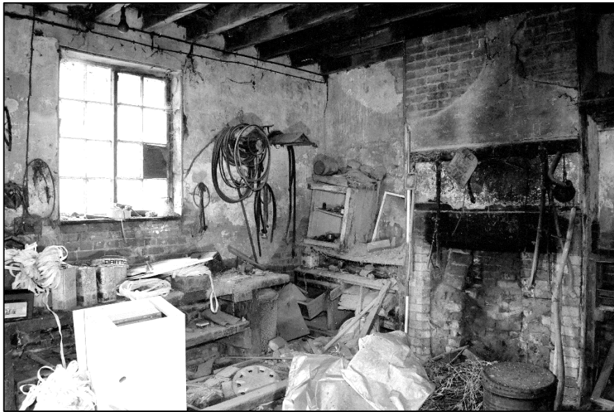
Appendix 2.30: View of the interior of Room G2, Building A , looking south-east
