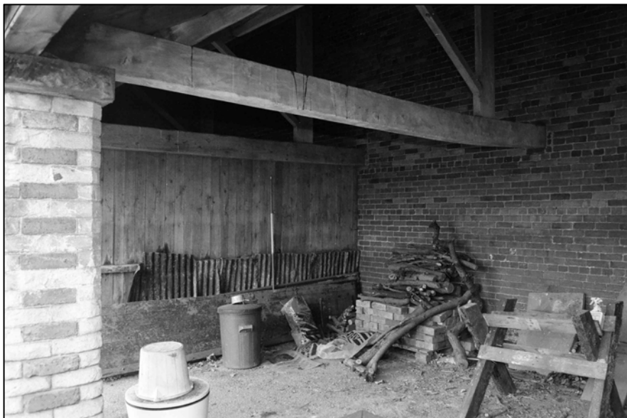
Appendix 2.35: View of the interior of Room G5, Building A , looking north-east
