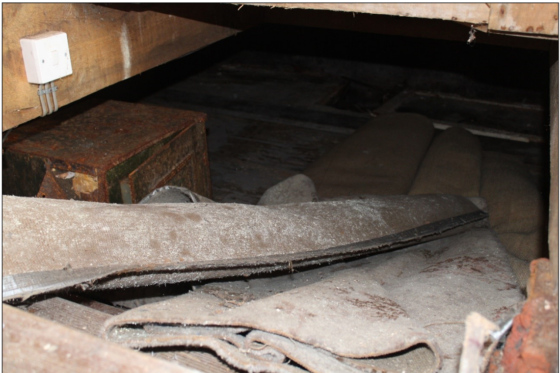
Plate 12: View under hatch in Room G2.
