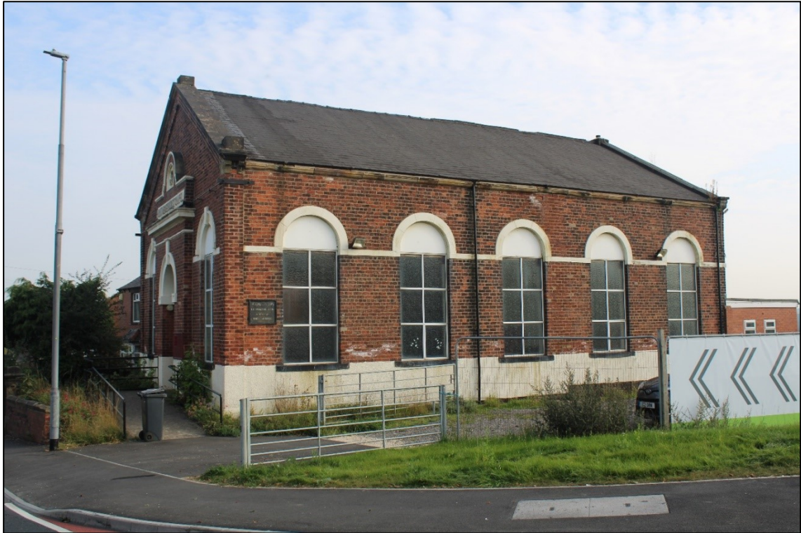
Plate 3: South facing elevation of the Barugh Methodist Chapel.
