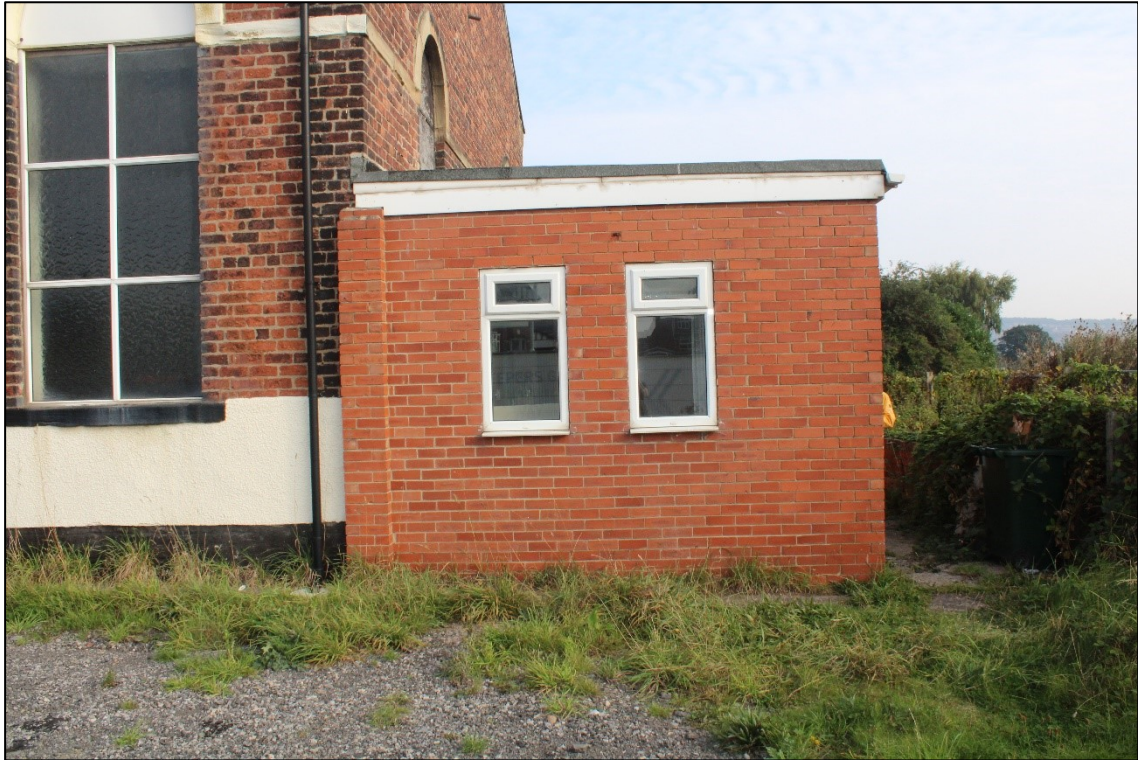
Plate 5: Detail of 1970s extension.
