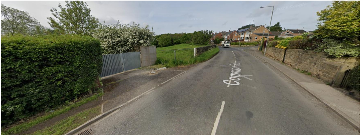
Image showing existing dropped kerb and proximity to bend on common road.
