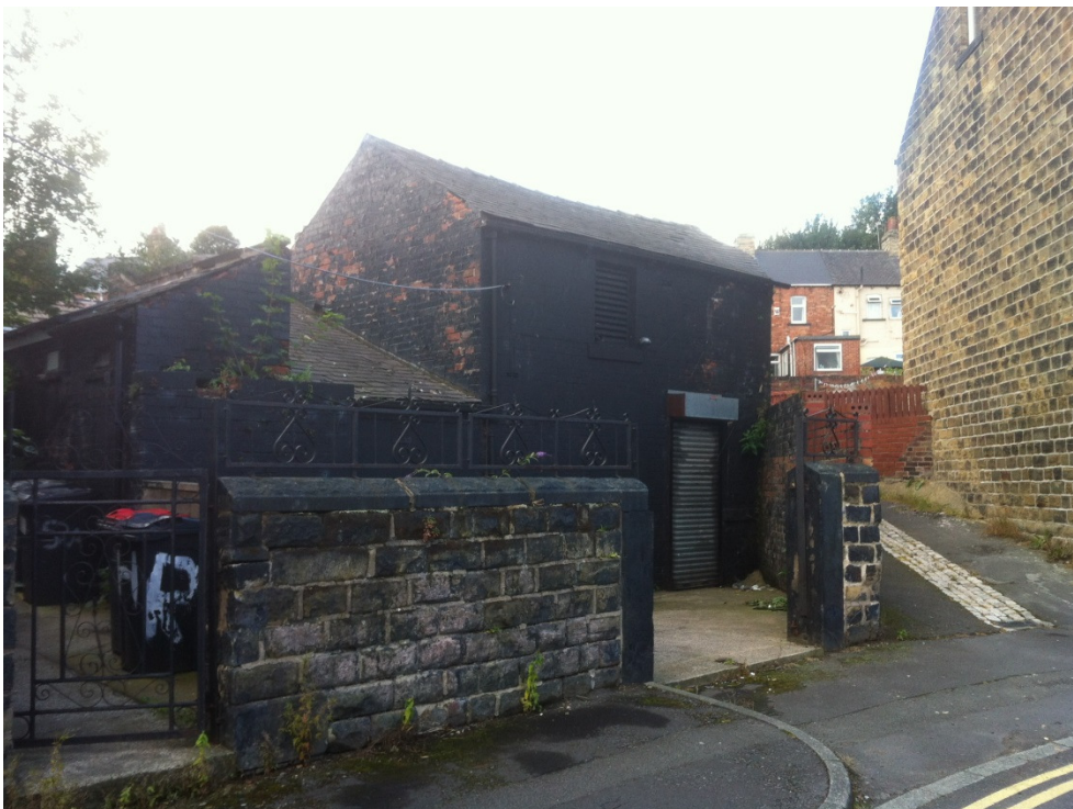
Fig 1. Existing building viewed from Honeywell Street
