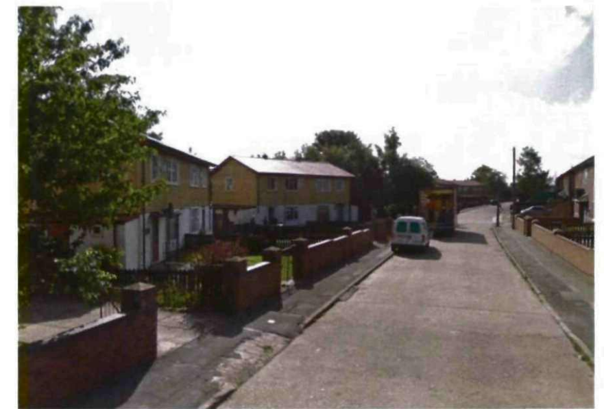
3. Southern view along Kirkstall Road showing properties which are now demolished.
