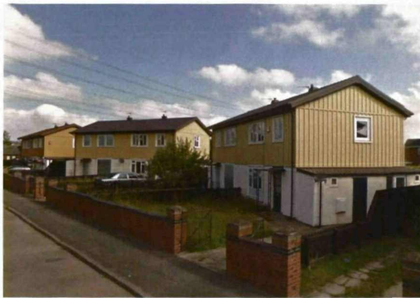
1. Northern view of now demolished properties along Kirkstall Road.
