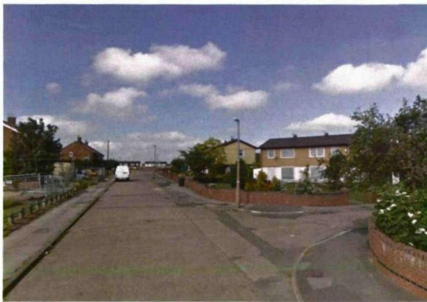
Southern view along Langsett Road showing properties which are now demolished.
