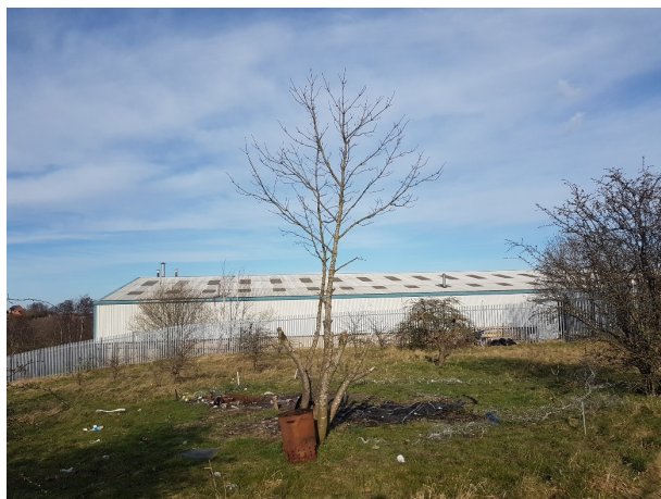
Photo 7: T23 from south west
