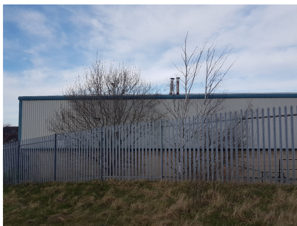
Photo 12: T41 and T42 from south west
