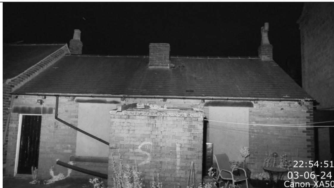
Photo 2 View from the rear (west aspect) of Building 1 – Canon XA50
