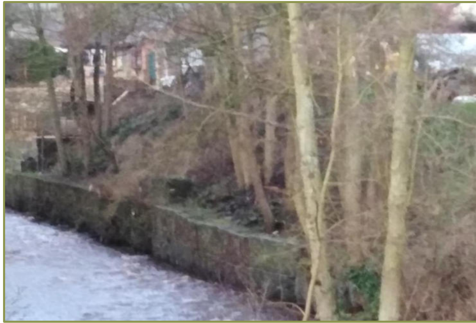
View looking north-west from Forge Lane Bridge towards the scrubland/woodland (Blue line Boundary) to the south of the Site
