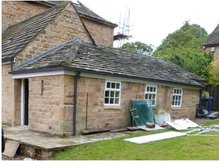
Figure 7 the linear extension to be demolished. The stonework changes surrounding, and below, the windows. These are clearly modern, inserted (c.1980) into older stonework that survives only at the ends with quoined angles – see also fig. 11. N.B. The lawned area before the single-storey outbuilding forms Zone 3 of the Hall's curtilage
