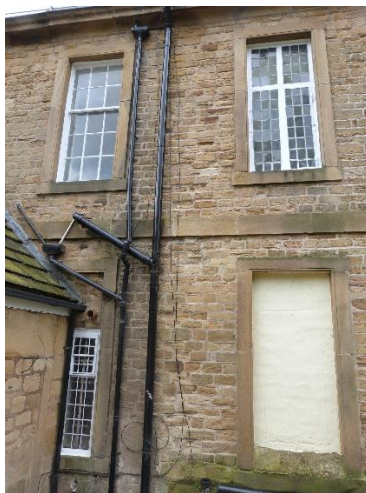
Fig. 12 north side elevation of house showing ground-floor blocked window and closer view of 1 st floor windows. The unsightly pipes have now (apparently) been removed and replaced internally.
