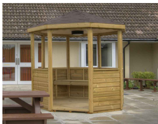
Smoking Shelter to Main Gardens
