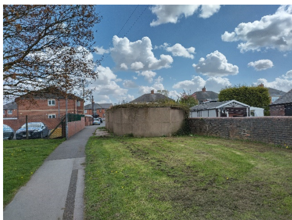
Photo 3: Site from northwest
