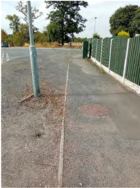
7 - scar which will be taking considerable loadings from delivery's
