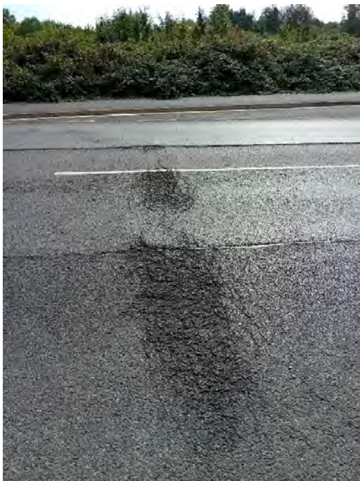
11 - crocodile patches which will get worse over time.
