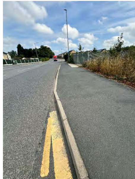
38- End of layby- good condition
