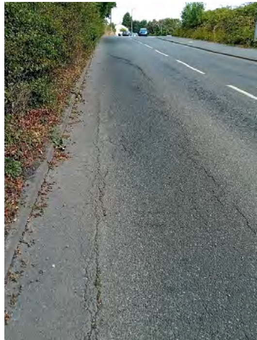
18 - Another angle looking back up towards derry grove junction
