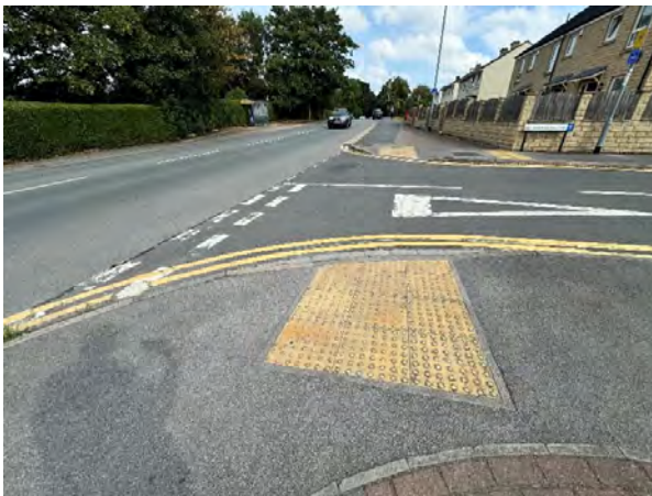
47 - Both tactiles in good condition
