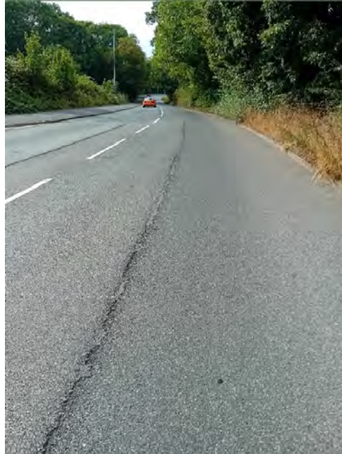
16 - another photo from root possible root damage
