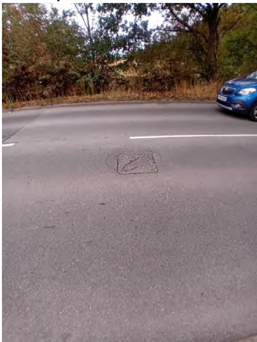
19 - Manhole lid in wheel line, in poor. 20 - Manhole lid in wheel line, in poor condition.
