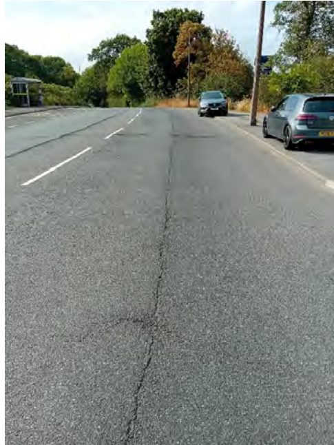
10 - jointing cracks
