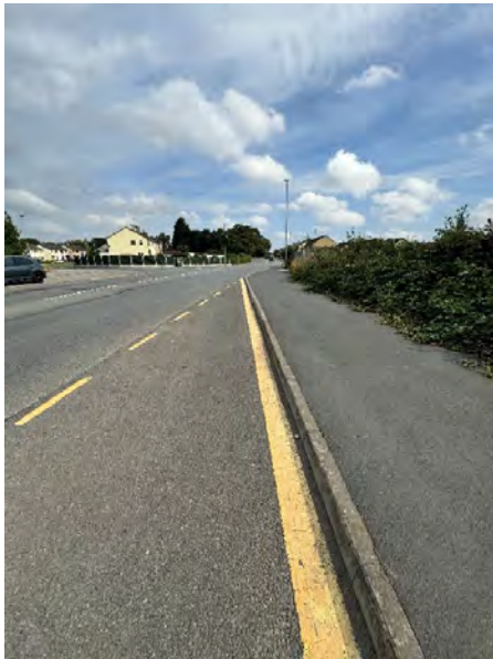
37- Bus layby Good condition
