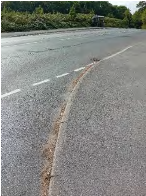
11 - crocodile patches which will get worse over time.
