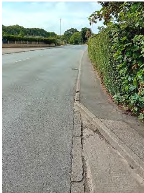
4 - Gully in good condition before radius to junction into site.
