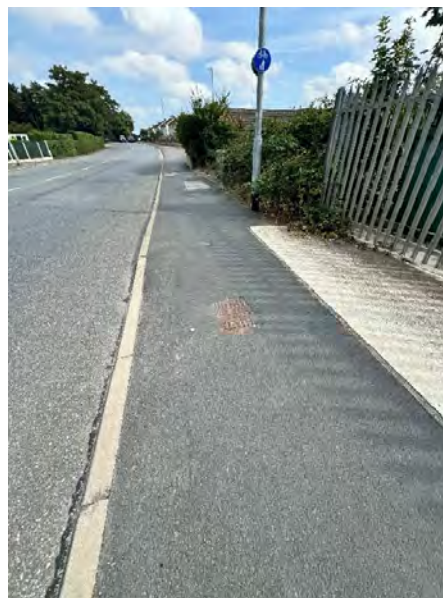
40- Manifold in good condition
