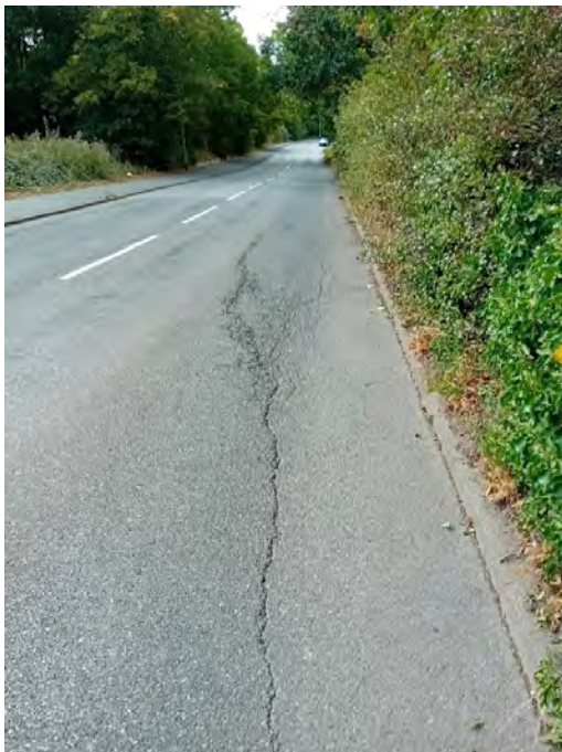
15 - potential root damage from mature trees in the verge
