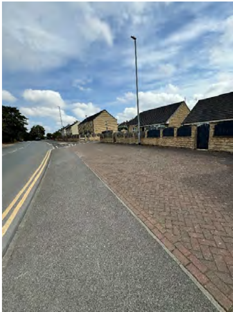
45 - Block paving/footpath in good condition .
