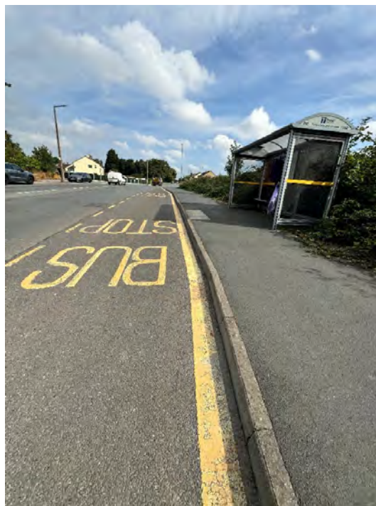
36 - Bus layby -good condition
