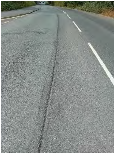
15 - potential root damage from mature trees in the verge
