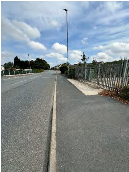
39 - Footway opposite DG Good condition .
