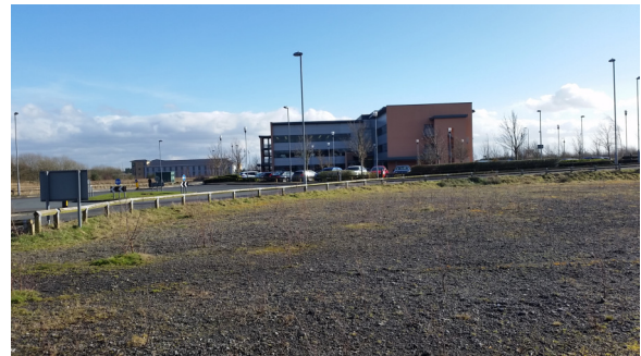
View looking south east to existing office building
