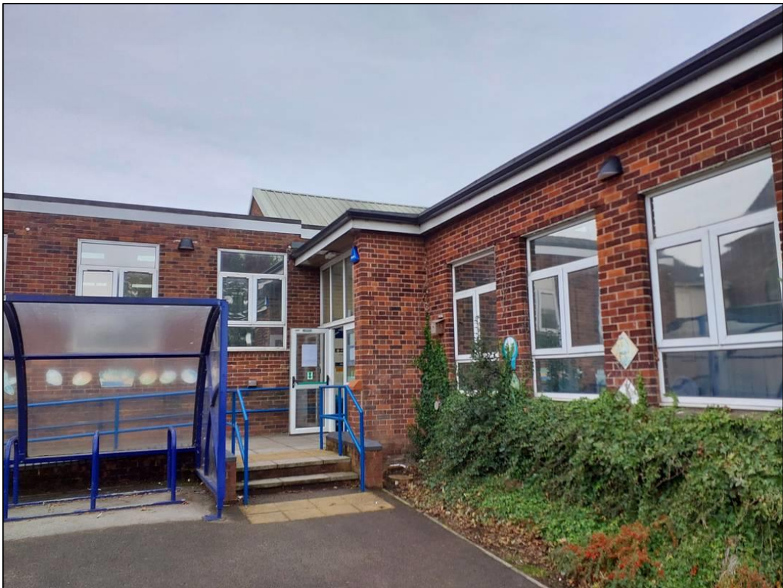
Photograph 4: Building 1 and introduced shrub
