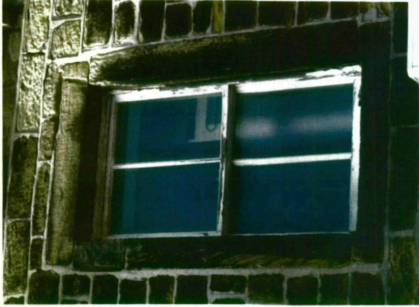
TYPICAL WINDOWS. GLAZING BARS - 25 mm thick. single glazed
