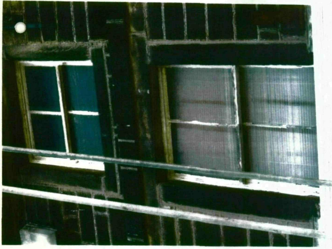
TYPICAL WINDOWS. GLAZING BARS - 25 mm thick. single glazed
