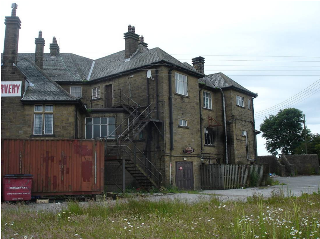
10. Rear elevation - north east, looking north.
