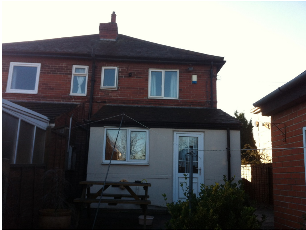
Fig 1. Rear elevation and adjacent extensions
