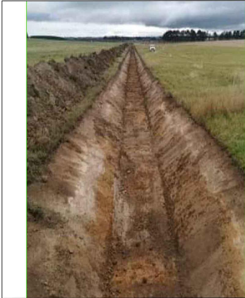
ILLUSTRATIVE PHOTOGRAPH OF DRAINAGE CHANNEL & BUND
