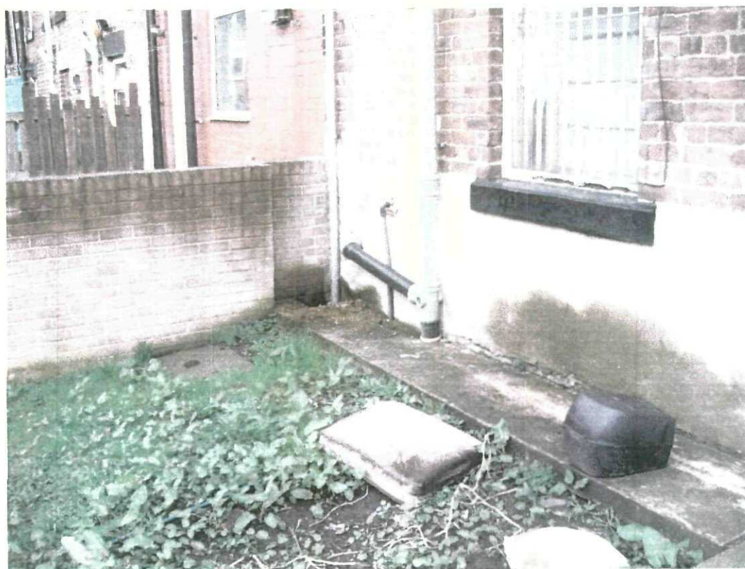
Figure 6 – View of Neighbouring property to East Boundary
