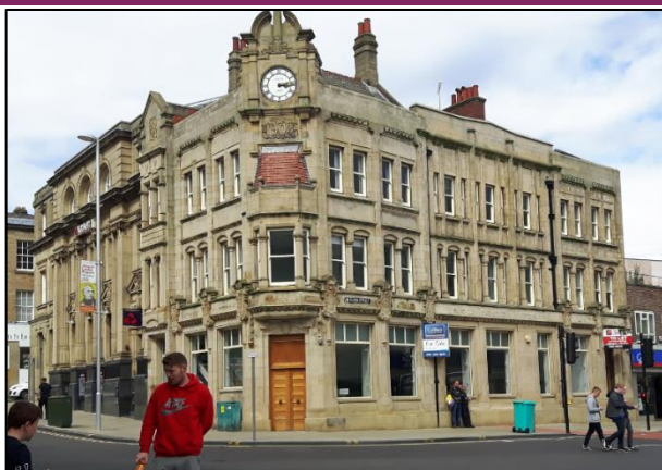
Image 1: 30 Market Hill / 2 Eldon Street, Barnsley (application site)
