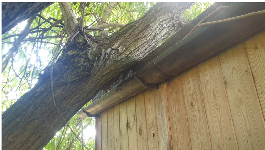
Photo 5: Large southern limb of T4 in contact with adjacent shed
