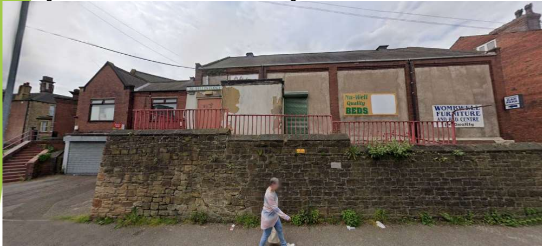
Existing site – rear view of the building facing East
