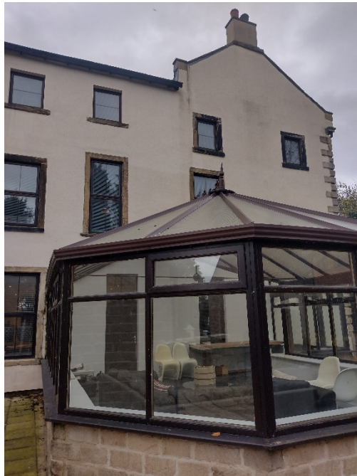
Fig 15: Existing splay ended conservatory and octagonal hipped roof incongruous against gable ends of principal heritage asset.
