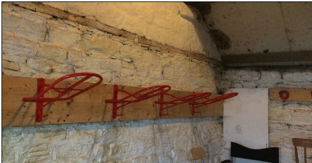
Inspection of large barn
