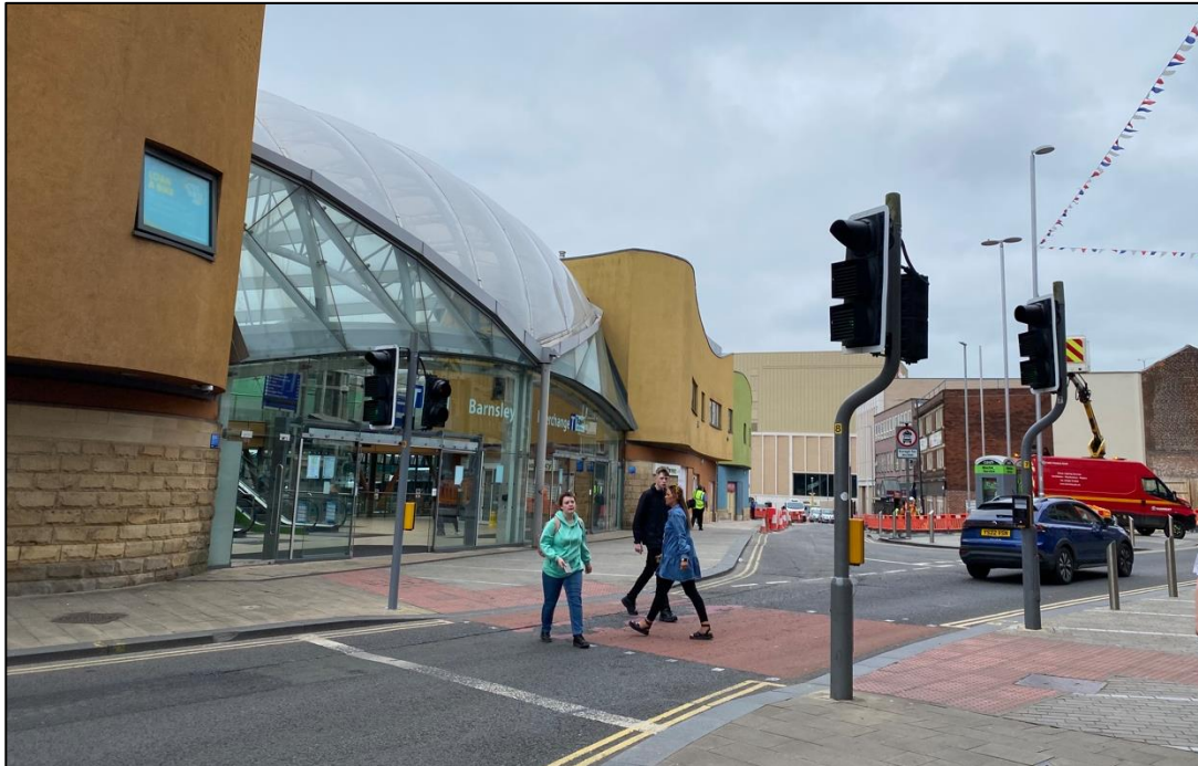
Figure 4-2 Barnsley Interchange pedestrian crossing
