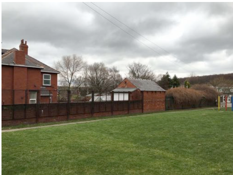
Figure 5 – View of North West Boundary to adjacent property
