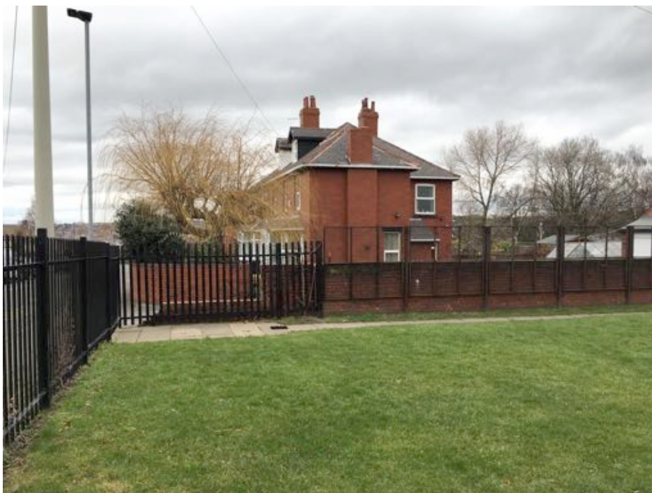
Figure 4 – View of North West Boundary to adjacent property
