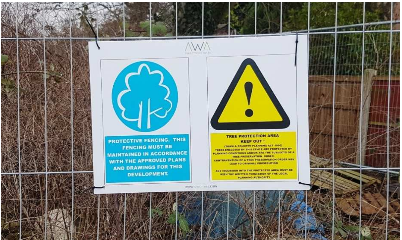
Figure 3: Example of A3 Correx Tree Protection Warning Sign fixed to fencing panel
