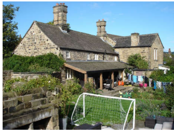
Fig 03. Chantry House East (rear)
