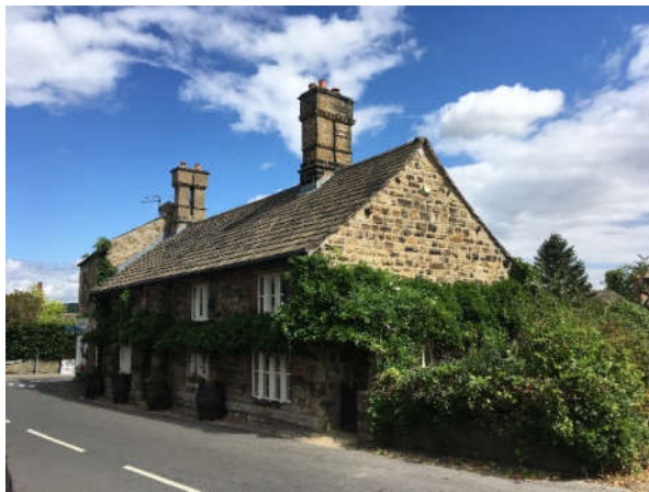
Fig 02. Chantry House South and West
