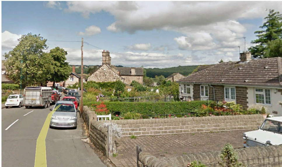
06. Photo from Church Street looking north showing gable wall of Chantry House.
