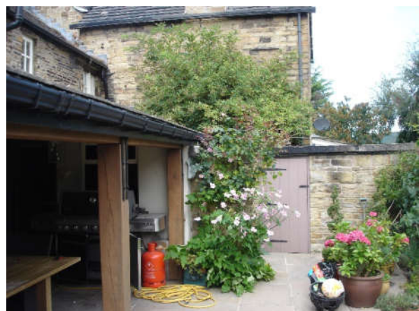
Fig 05. Canopy and flat roof outbuilding.
