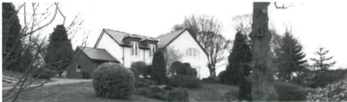
Newly constructed rendered dwelling
