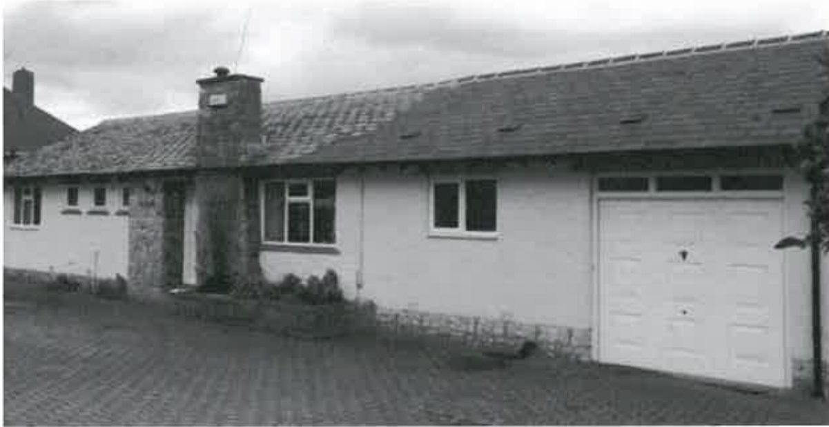
Photograph of front / east elevation
