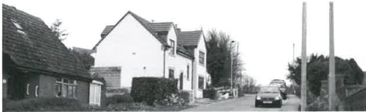
Newly constructed rendered dwelling
