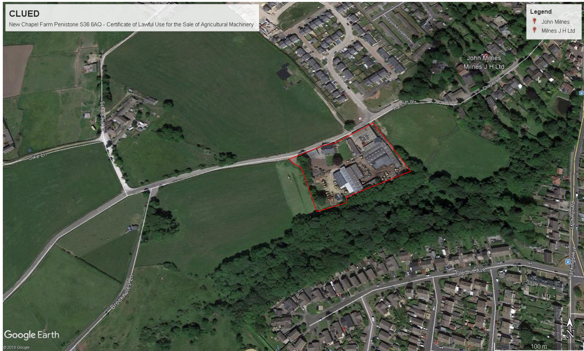
Aerial Photograph of May 2017 showing the machines parked by south side boundary in a line ready for repair, painting and cleaning in the workshops.
