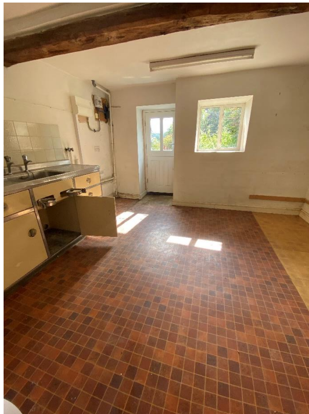
Figure 7 Existing dated kitchen area.
