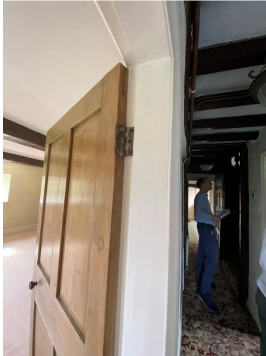
Figure 48 Showing the hallway passage. The beams are exposed to the hallway and covered over in the living room.
