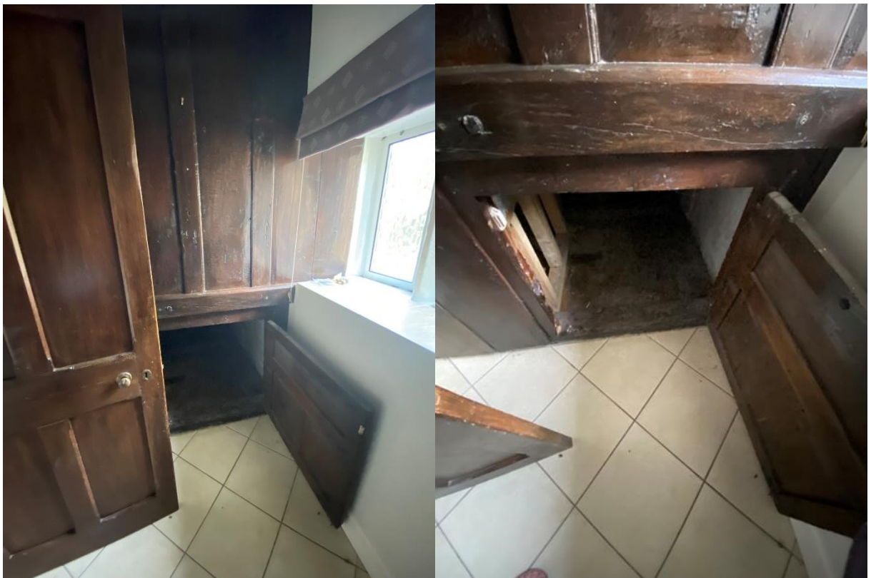
Figure 51 Original understairs cupboard in bathroom.
