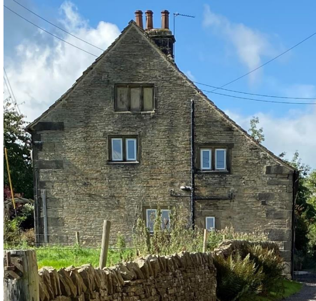
Figure 22 C17 Northeast elevation, showing blocked up three light window in the loft area. Ashlar chimney stack to the roof.
