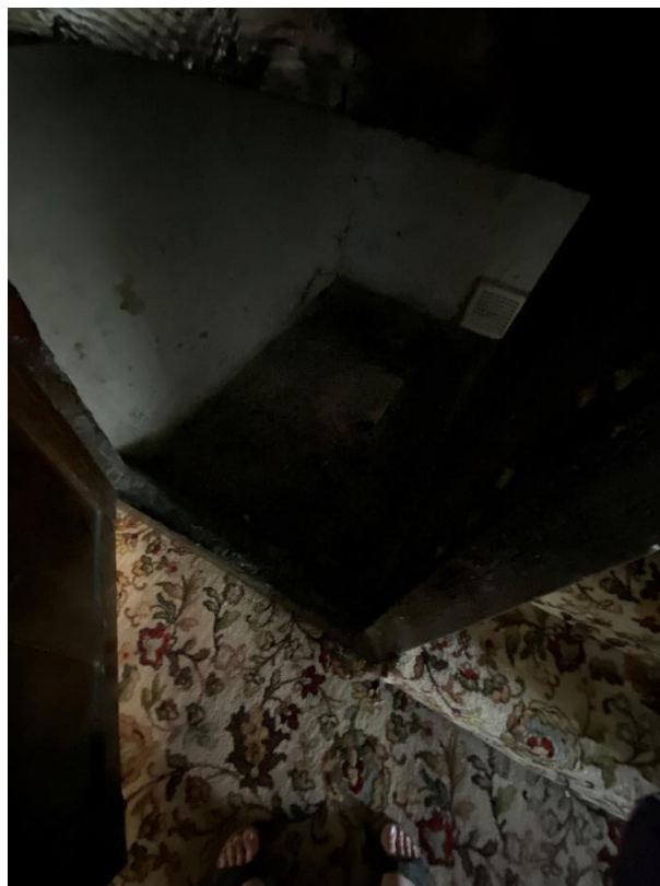
Figure 53 Showing inside the understairs cupboard, with modern air vent inserted into outer wall.
