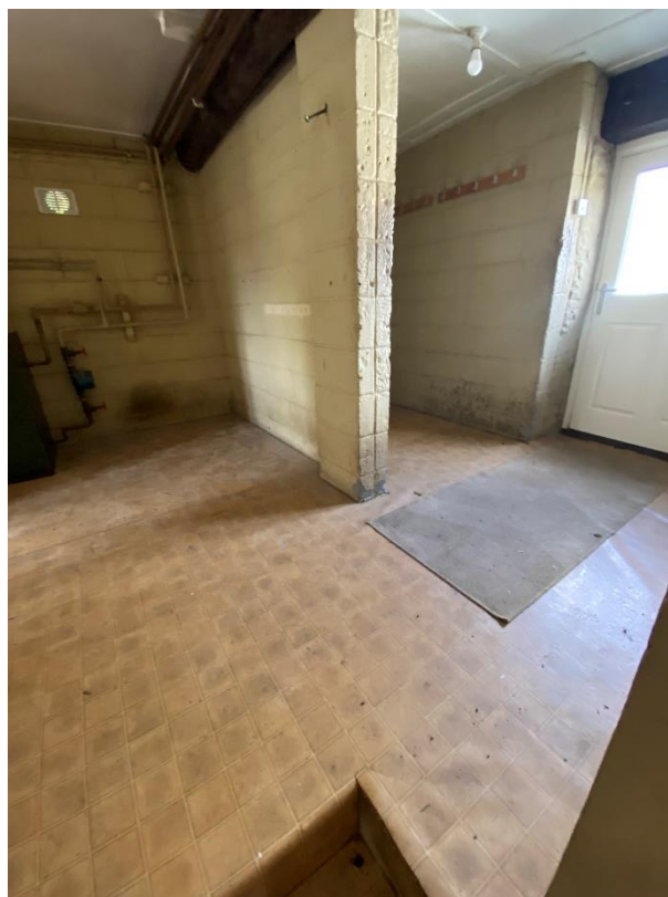
Figure 35 Showing the entrance from the northwest elevation into the lobby/boot room. Original beam to the ceiling.
