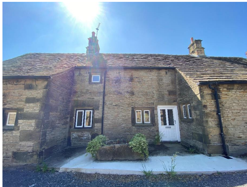
Figure 23 Showing the C17 northwest elevation, doorway was on the left hand side originally.
