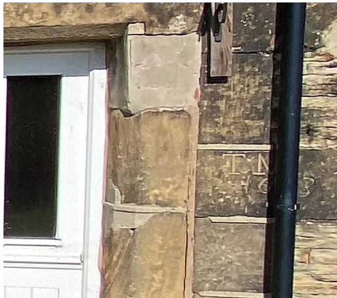
Figure 31 Detail of the inscription of quoin stone "TM 1693". Also evident is repair to the stonework around the door.
