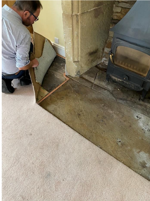
Figure 46 Showing floorboards next to the hearth in the living room.
