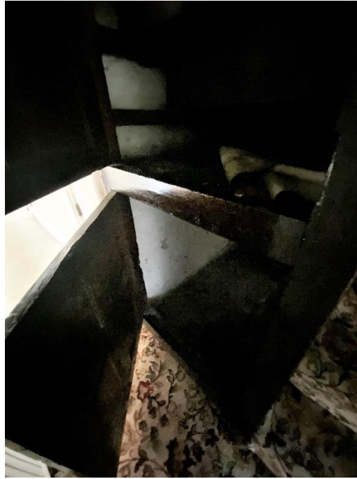
Figure 54 Showing inside of the understairs cupboard showing signs of damp and needs attention.
