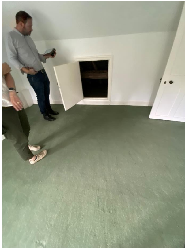
Figure 64 Bedroom 1 eves storage.
