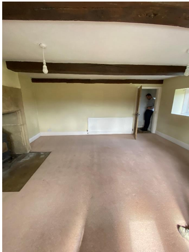
Figure 47 Showing doorway in living room into the hall way passage. This looks to be a partition wall with insert door added.
