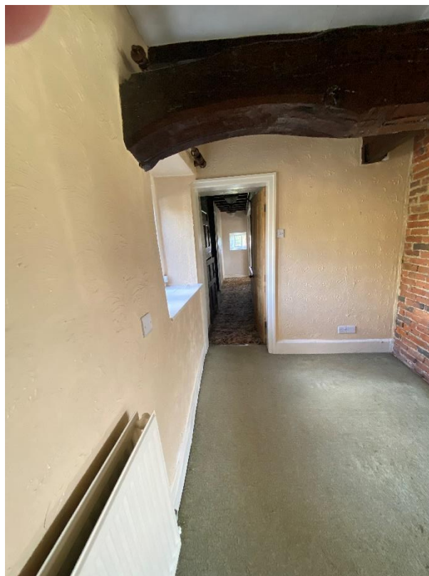
Figure 43 Showing the bressumer beam carved out for headroom. This was the original entrance into the sitting/dining room where the window now is. See next figure for an example of how it could have been originally.
