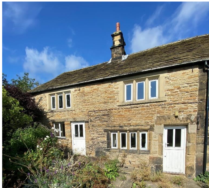
Figure 29 Southeast elevation of the later addition. Window cills, lintel, and mullions to the first floor appear to be replacements.
