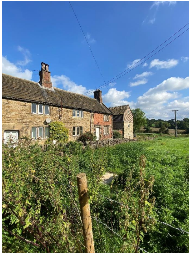
Figure 17 Showing the Front facade of Jowett House and adjoining cottage.
