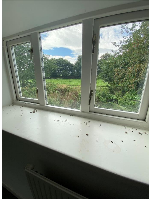
Figure 28 View from the southwest elevation first floor window.
