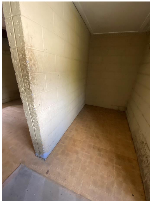
Figure 33 Breeze block dividing wall in the lobby/boot room.
