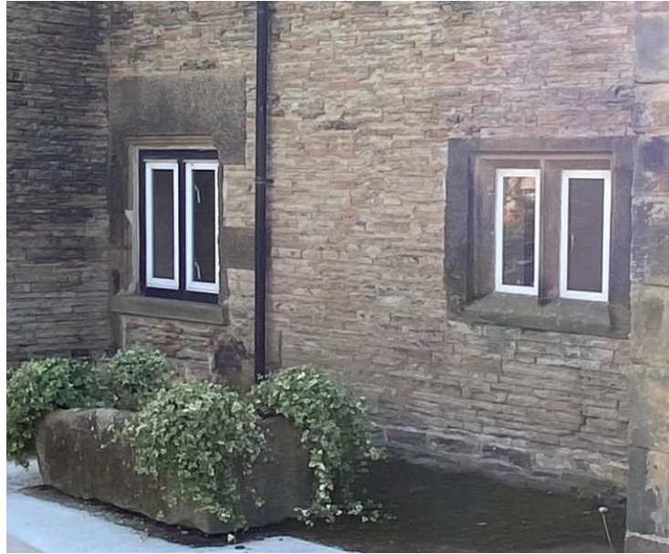
Figure 24 Detail of the former doorway on the left within the C17 northwest elevation.
