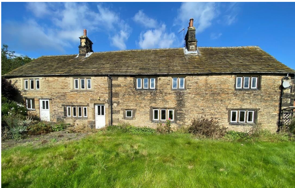
Figure 16 Showing the southeast elevation of the house the right-hand side dated to C17.
