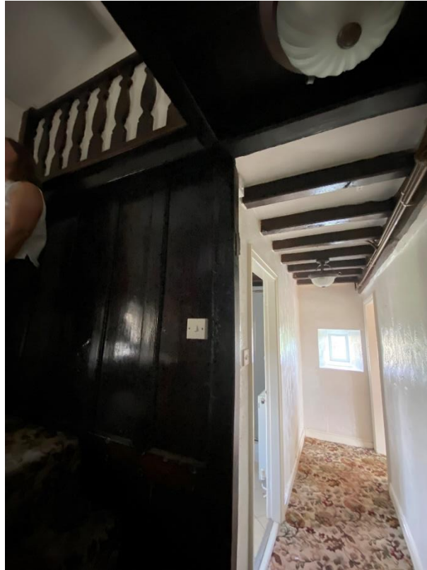
Figure 52 Original joinery of the staircase, possibly would have been an open balustrade into the eaves.
