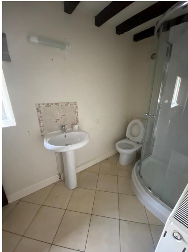
Figure 50 Downstairs bathroom with original beams.
