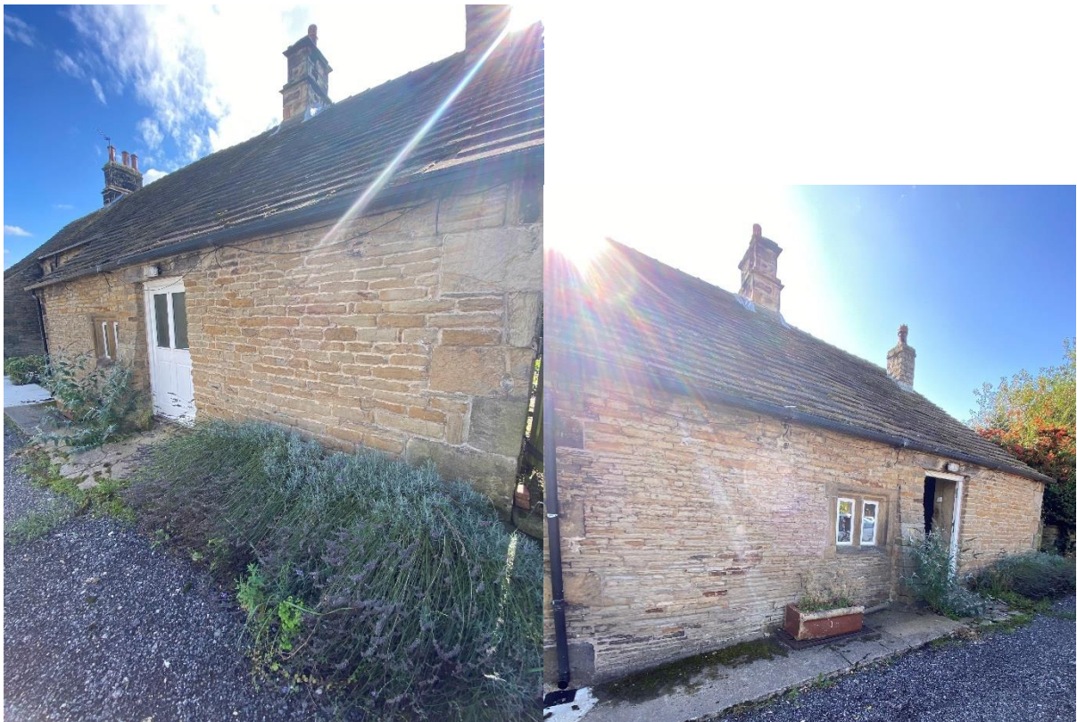
Figure 25 Two images showing the northwest elevation of the later addition with Ashlar chimney stack and brick chimney stack.
