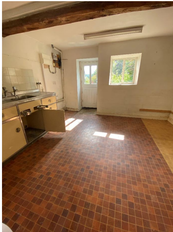
Figure 36 Showing the utility room and entrance out to the garden. Original beam to the ceiling.
