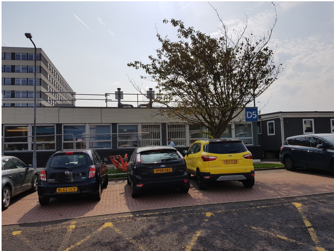
View of North East Elevation – Western End
