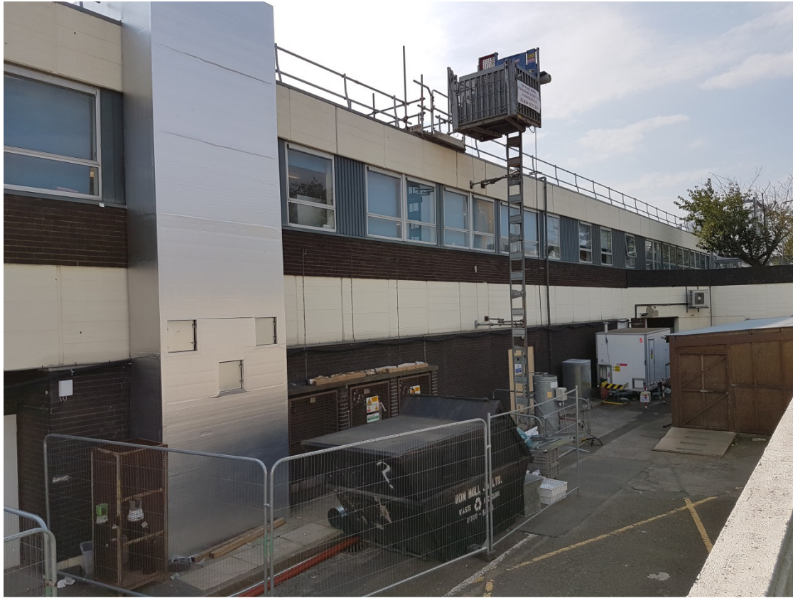
View of North East Elevation From The East
