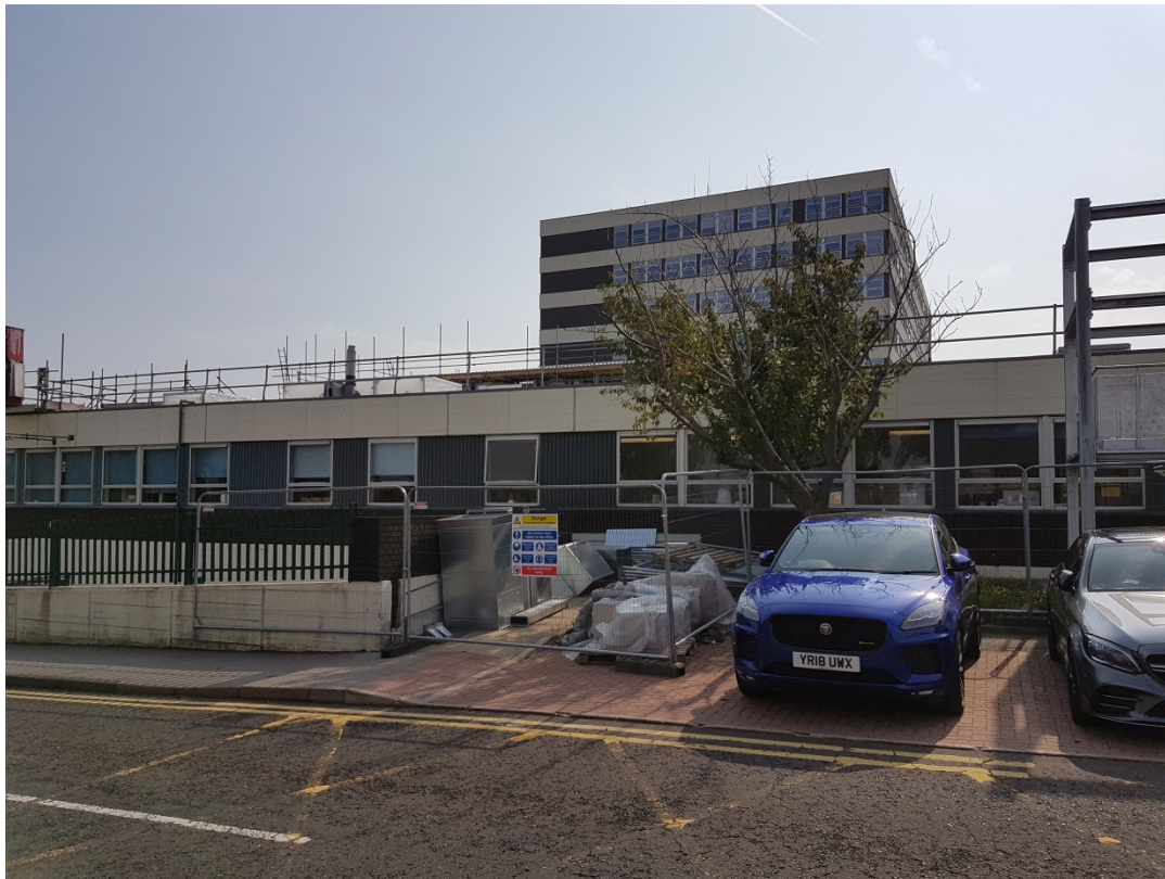
View of North East Elevation – Eastern End
