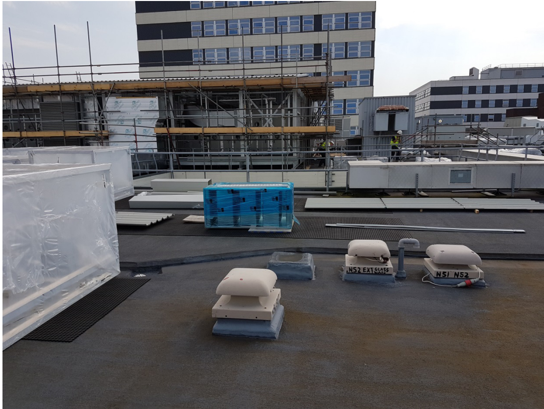
View of Proposed Site Looking South
